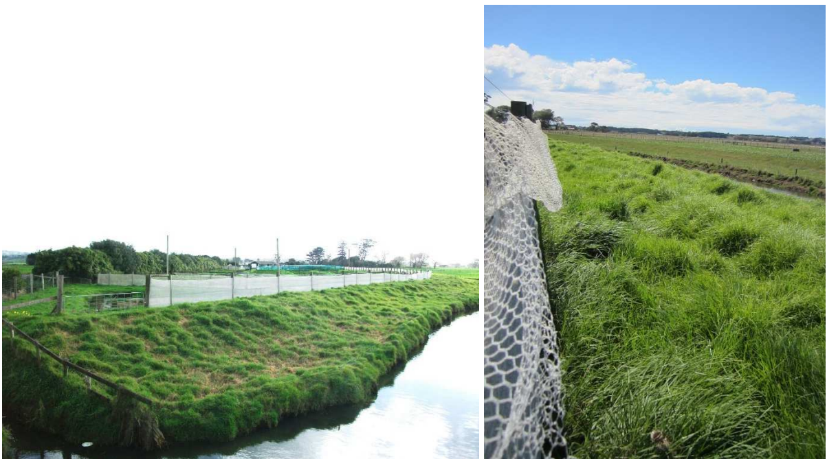
Figure B29. The eastern boundary of the site showing the mesh fence on the earth bund beside the canal (Left, photo by S Pullan, August 2013), and a close-up of the mesh fence (right, photo by J Clayton, March 2014).
