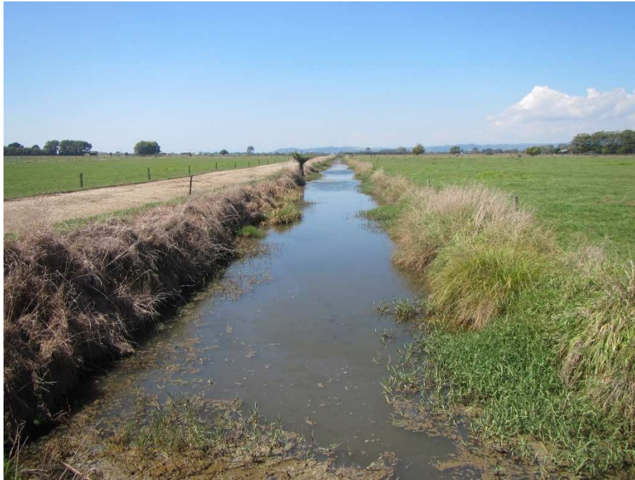
Figure B5. Massey drain approximately eight weeks post spray with herbicide. The drain is largely weed free but there were some patches of dense weed growth (in the distance).
