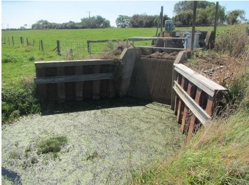
Figure B7. Awaiti East drain showing fragmented C. demersum that had collected at the screen.
