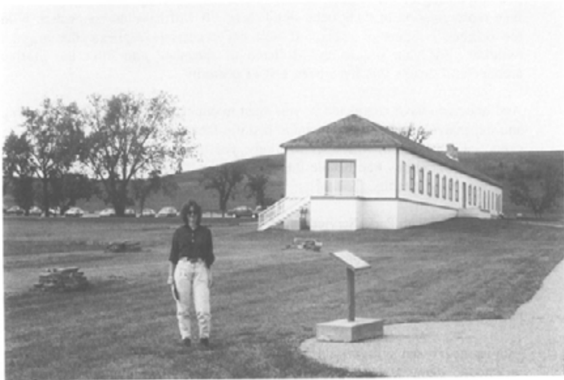
Figure 11 Reconstructed commissary and Civilian Conservation Corps outline of barracks (foreground). The reconstructed building is placed on a steel framework on caissons (large steel pipes), while the excavated archaeological site beneath is protected by an earth pad about one metre thick. Note sign on concrete footing, not dug into ground.
