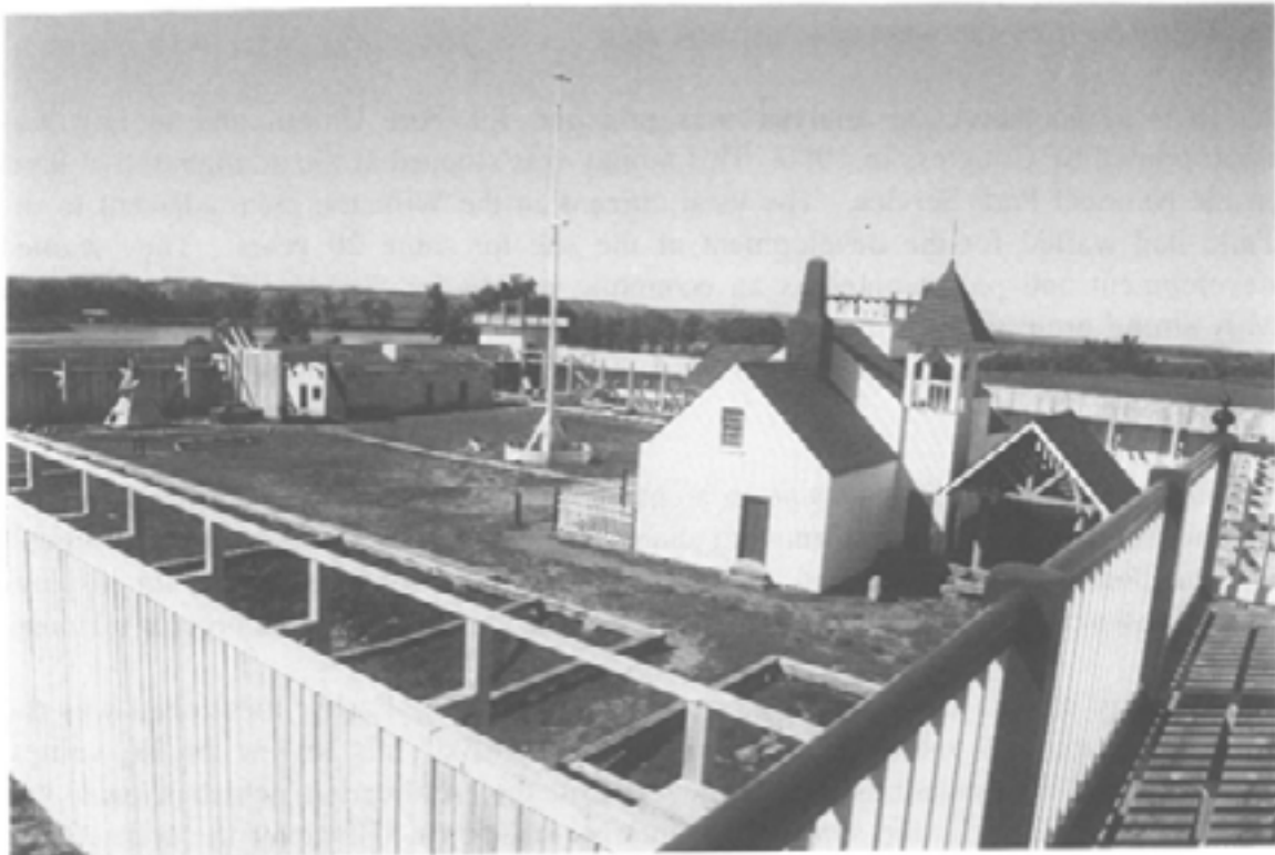
Figure 8 Fort Union Trading Post National Historic Site from the tower of the north-east bastion, the Bourgeois's House centre right. To the right of the Bourgeois's House is a protective roof for the exposed kitchen foundations. The stockade and internal wooden bracing run out to the left. The outlines of the "barracks" within the walls are marked by horizontal wooden beams. By the entrance, centre left, is the earth-roofed trade house.
