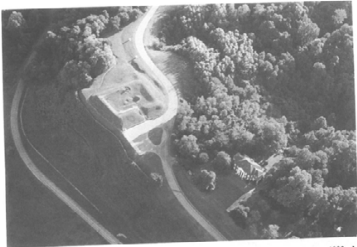
Figure 26 Fort Hill, in the north loop of the Vicksburg National Military Park, September 1993; the view is to the northeast. A concrete surface drain has been installed along the steep slope (at left, in shade) about 10 m down from the crest, to stabilise the edge of the bluff. Note house in the immediate park vicinity, lower right.
