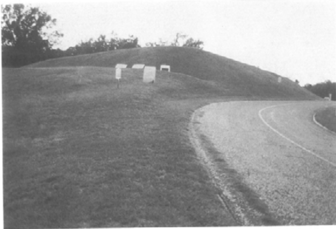
Figure 25 Stockade Redan in September 1993, from a similar vantage point to Fig. 24. The redan is as restored by stabilisation programmes in the early part of this century.
