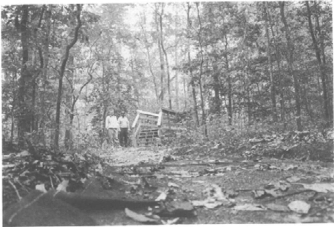
Figure 38 Track details at Cold Harbor, Richmond National Battlefield Park, Virginia. The track is gravelled over a slight excavation covered by a geotextile. The geotextile prevents mixing of the gravel and subsoil, while allowing free drainage. Where the track crosses the Union lines, a footbridge has been erected.
