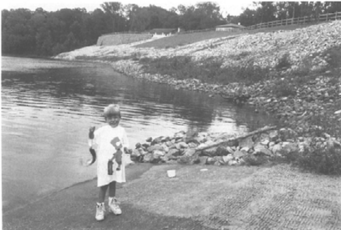
Figure 23 Rip-rapped slope, Moundville Archaeological Park, near Tuscaloosa, Alabama. The Black Warrior River cut into the alluvial soils threatening the convention centre, centre top, and the site beyond. All rip-rap and machinery was brought in by barge on the river, avoiding damage to the wider archaeological site.
