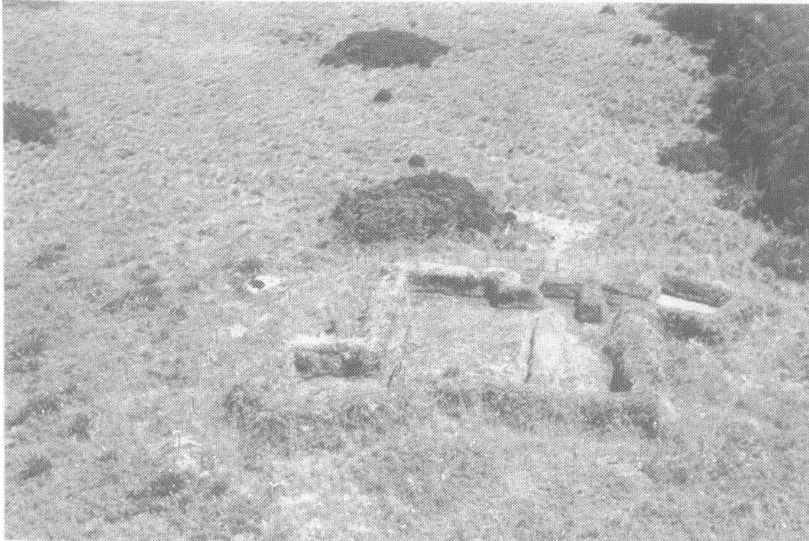
Figure 37(e) Aerial view of Te Porere upper redoubt (T19/55) from the east in about 1961 after restoration by the late Ormond Wilson and team. Note bulge (overhang) and cavity in base (both marked by shadow) in far wall. Photo credit: New Zealand Historic Places Trust.
