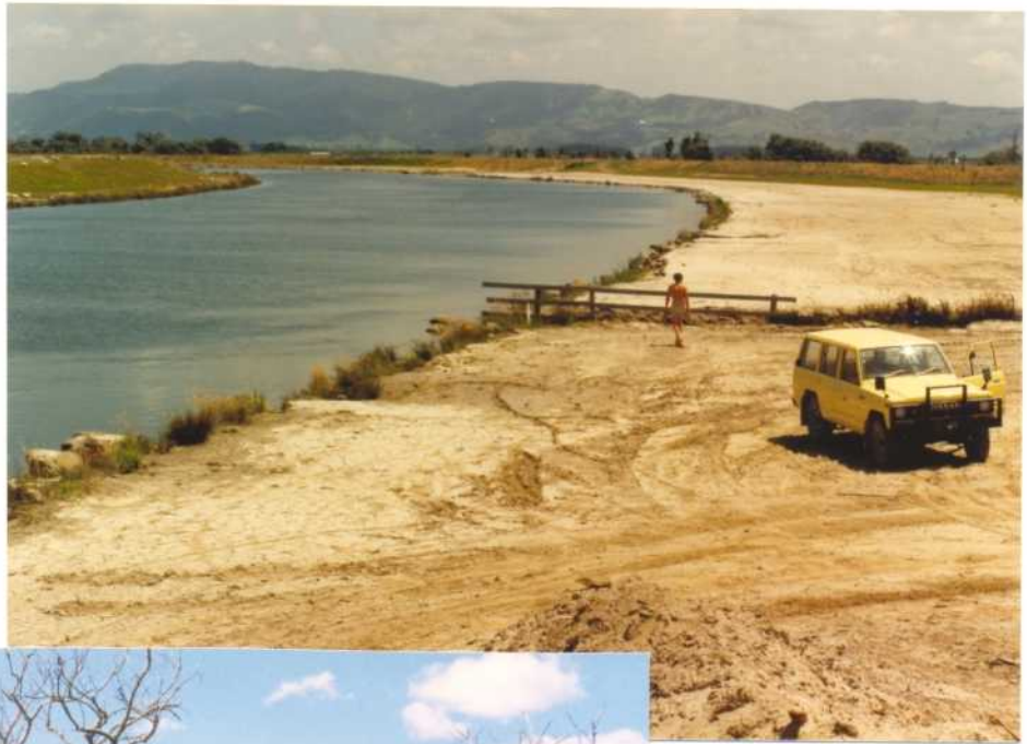
Figure 3 Grading the lower Kaituna River floodplain.
