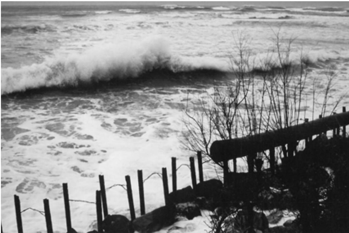
Plate 6 Southeasterly swells reflecting off a rock seawall at Wainui Beach, Gisborne, 1992. Breaking wave heights effectively doubled, exacerbating the erosion problem.
