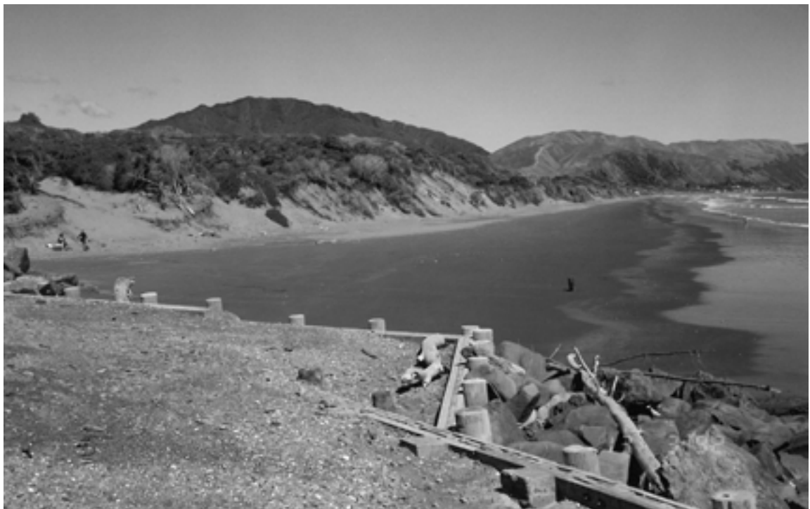
Plate 7 Looking south from the Raumati seawall, Kapiti Coast, 13 March 1992. Since 1974 the foredunes have retreated about 45m because of the seawall, coupled with a long- trend of retreat.
