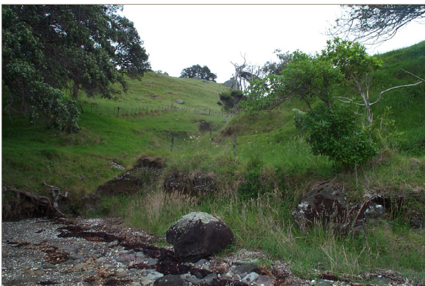
Figure 23. Coastal erosion at Q07/797 (around McGregors Bay, Whangarei Heads, November 2005).
