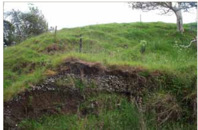
Figure 24. Changes to water table and flow can undermine land and create slumping and erosion, as shown at Q07/797, McGregors Bay, Whangarei Heads (November 2005).
