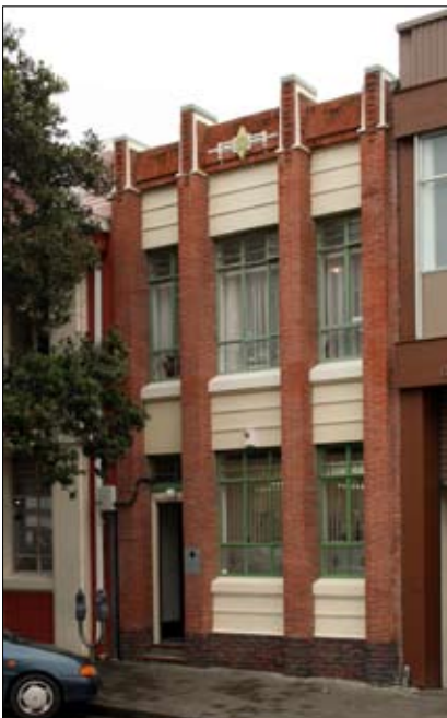
Figure 13. J.A. Louis Hay Office Building, Herschell Street, built 1932.
