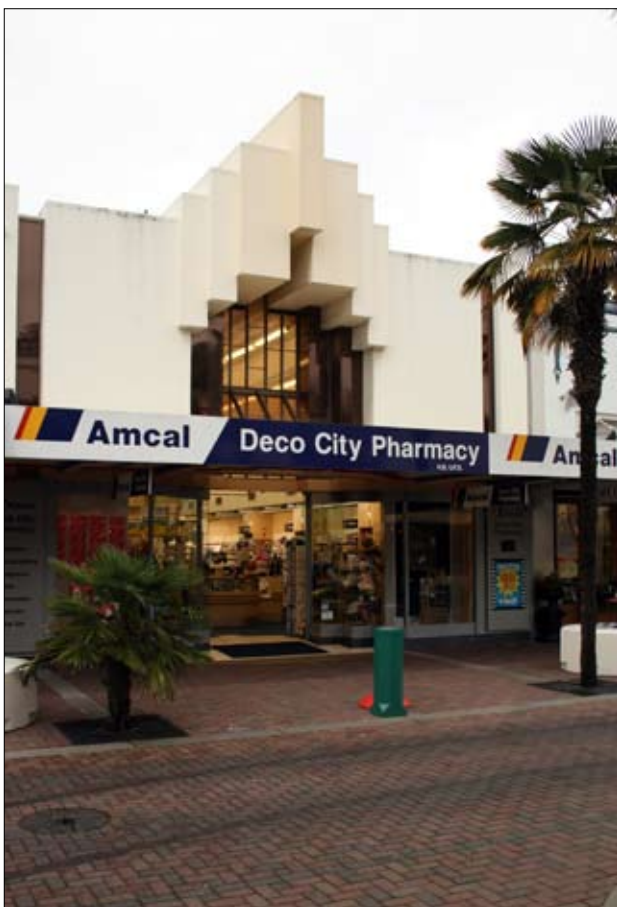
Figure 19. Amcal Pharmacy; an example of sympathetically scaled infill on Emerson Street.
