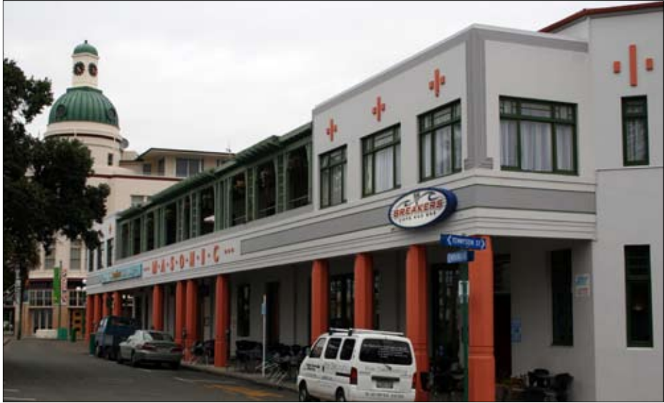
Figure 8. Masonic Hotel, Herschell Street, built 1932.
