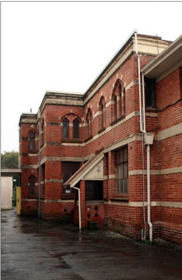
Figure 5. Diocesan Hall and Offices, Diocese of Waiapu, Cathedral Lane, built 1929.
