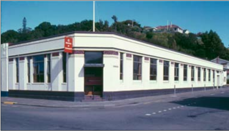
Figure 10. Ross & Glendinning Building, Tennyson Street and Cathedral Lane, built 1932.
