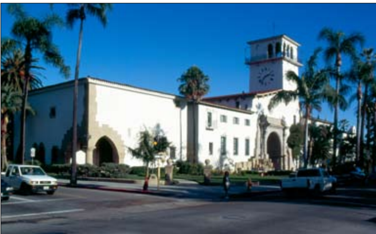
Figure 23. Santa Barbara County Courthouse, Santa Barbara, CA, built 1925–29.
