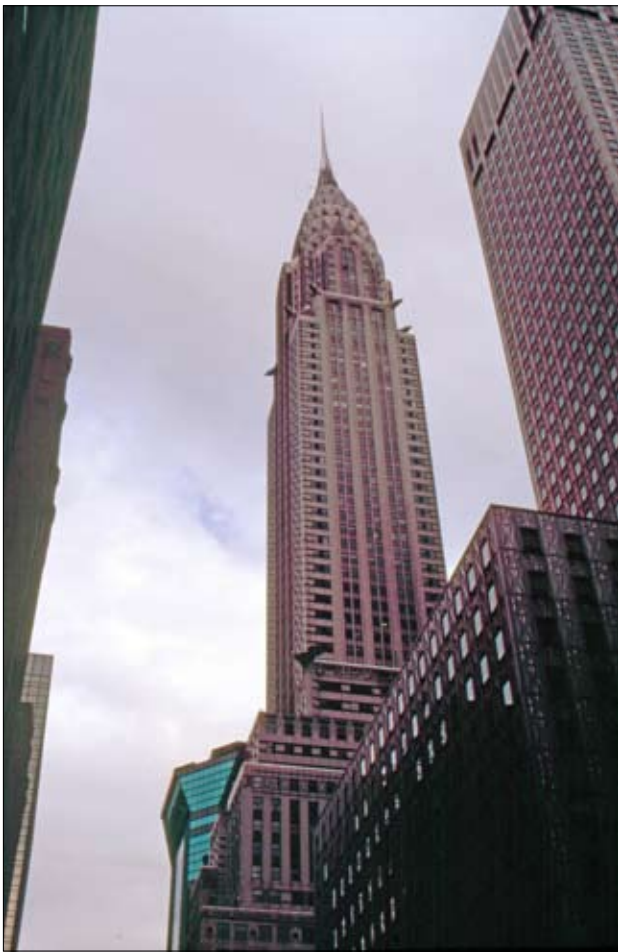
Figure 24. Chrysler Building, New York City, NY, built 1930.
