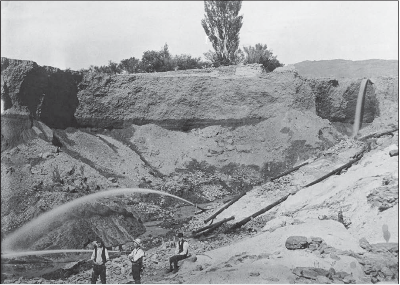
Figure 11. Sluicing, Hancock & Lawrence's Claim, Bannockburn (no date). Reproduced by courtesy of Hocken Library, Uare Taoka o Hakena, University of Otago.
