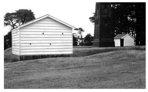
Figure 105. Manaia Redoubt: the Parihaka Campaign fortification has two blockhouses at opposite angles for flanking defence. A concrete tower at the centre of the square redoubt replaces the original wooden watch-tower. *Photo: N. Prickett, 1975.*
