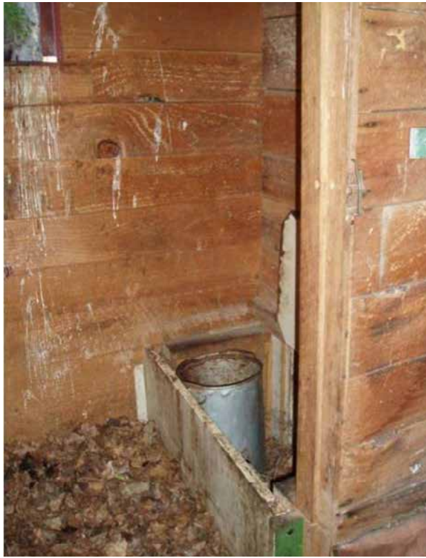
Figure 34. The can toilet in Room 5 of the Barkers' house. Photo: Katharine Watson.
