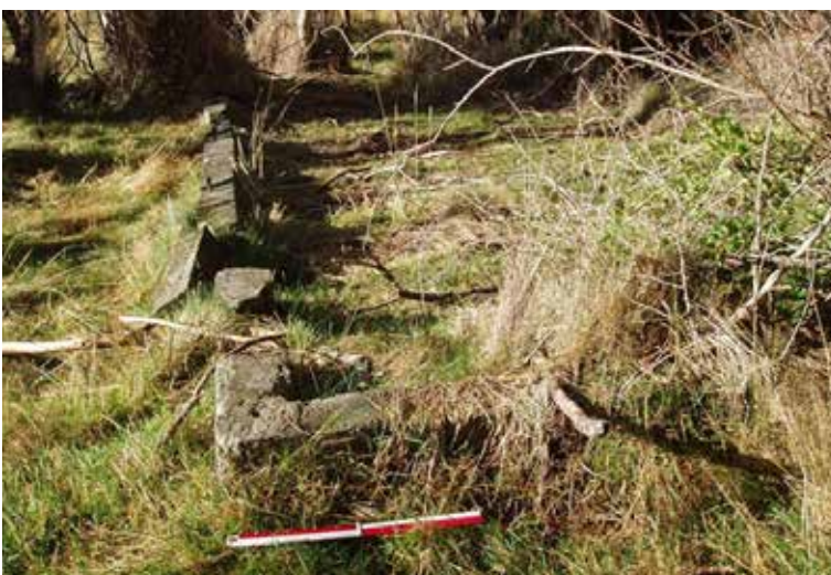
Figure 56. The concrete foundations of the refrigeration unit at the hockey rink. Photo: Katharine Watson.
