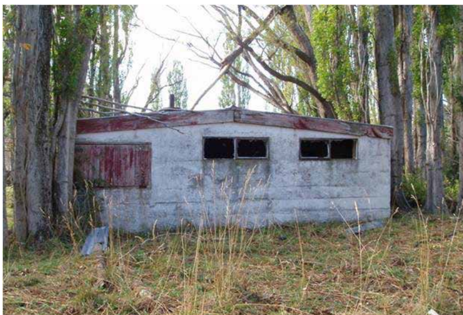
Figure 35. The west elevation of Phase 2 of the Barkers' house. Photo: Katharine Watson.
