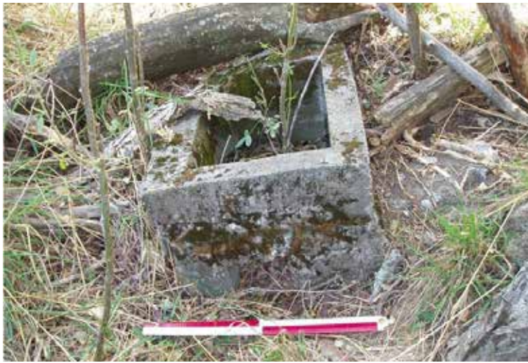
Figure 39. Concrete boxing associated with the house water race. Photo: Katharine Watson.
