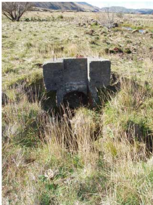
Figure 15. The concrete culvert and control structure. Photo: Katharine Watson.
