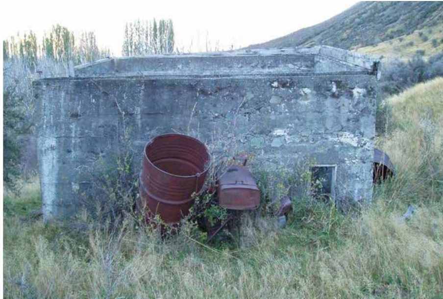
Figure 60. The power house. Photo: Katharine Watson.
