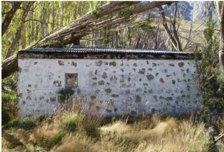
Figure 40. South elevation of the White Hut. Photo: Katharine Watson.
