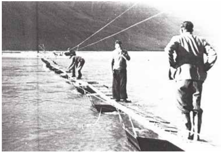
Figure 8. Crossing the Rangitata River on the pontoon bridge. Source: Geraldine Museum 1825 .
