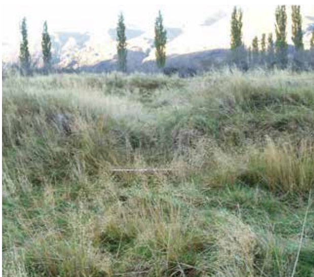
Figure 22. A gap in a bund to enable the flow of water between rinks. Photo: Katharine Watson.
