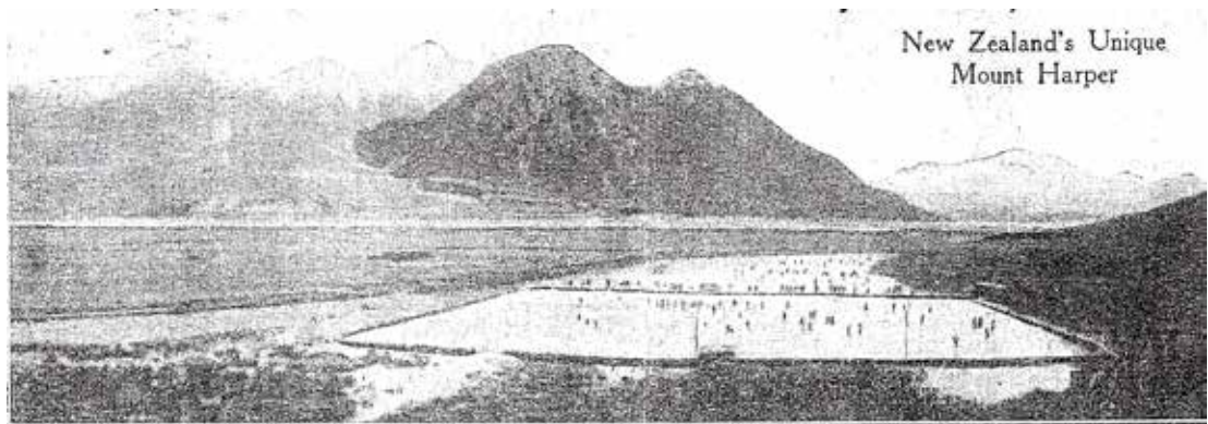
Figure 4. The Mt Harper ice rink in 1940, looking west. Source: The Press , 2 July 1940.
