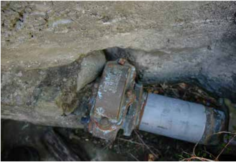
Figure 62. The overflow pipe from the power house. Photo: Katharine Watson.
