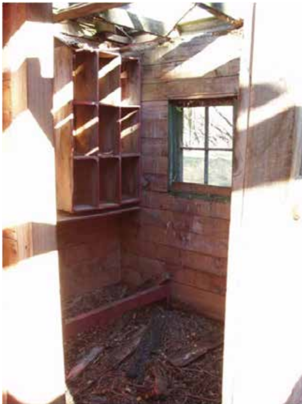
Figure 30. Storage space in Room 2 of the Barkers' house. Photo: Katharine Watson.
