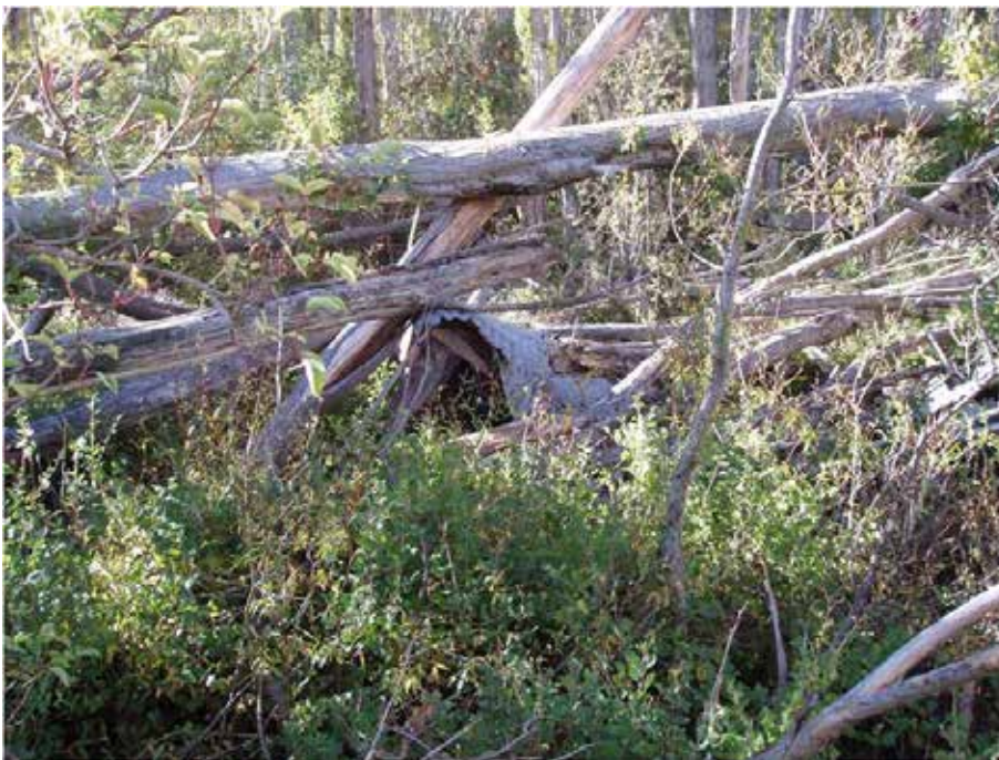
Figure 46. The collapsed remains of the hen house, near the White Hut. Photo: Katharine Watson.
