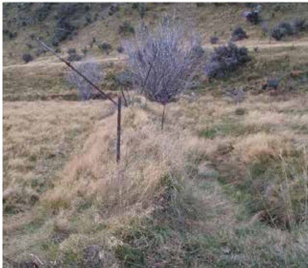
Figure 21. Power poles/lampposts along the bund on the east side of Rink 2. Photo: Katharine Watson.
