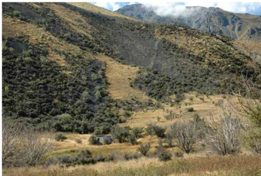
Figure 59. The power house (the concrete structure in the middle distance), clearly showing the route of the penstock down through the scree. The zig-zag track can just be made out to the left of this. Photo: Katharine Watson.
