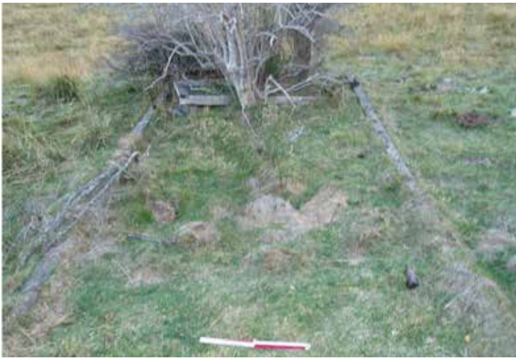
Figure 54. The foundations of the ticket office. Photo: Katharine Watson.
