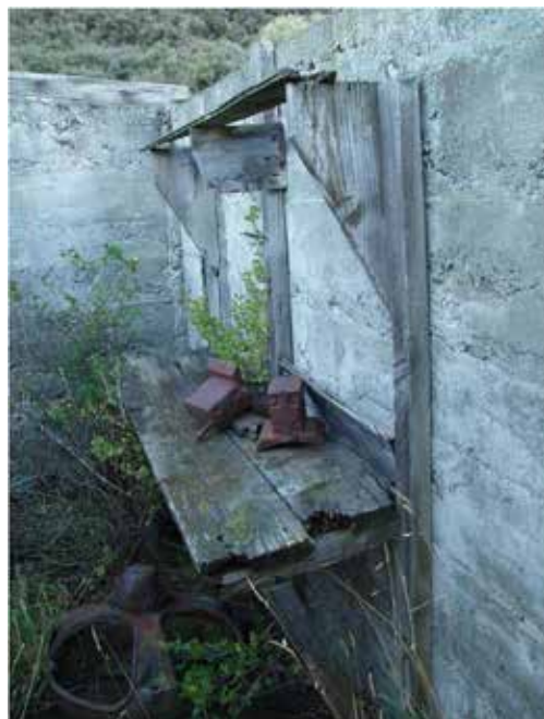
Figure 66. The in situ work bench in the power house. Photo: Katharine Watson.
