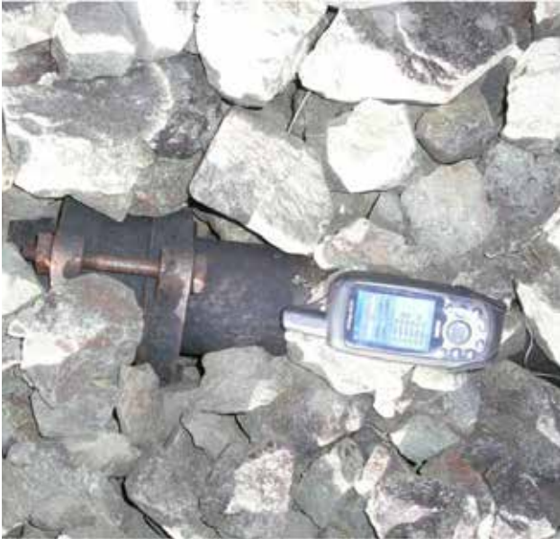
Figure 57. The penstock buried in the scree. Photo: Ian Hill.
