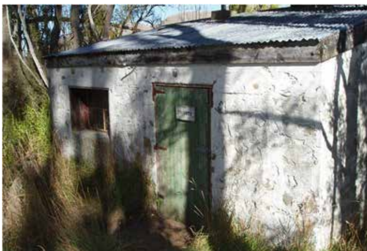
Figure 41. North elevation of the White Hut. Photo: Katharine Watson.
