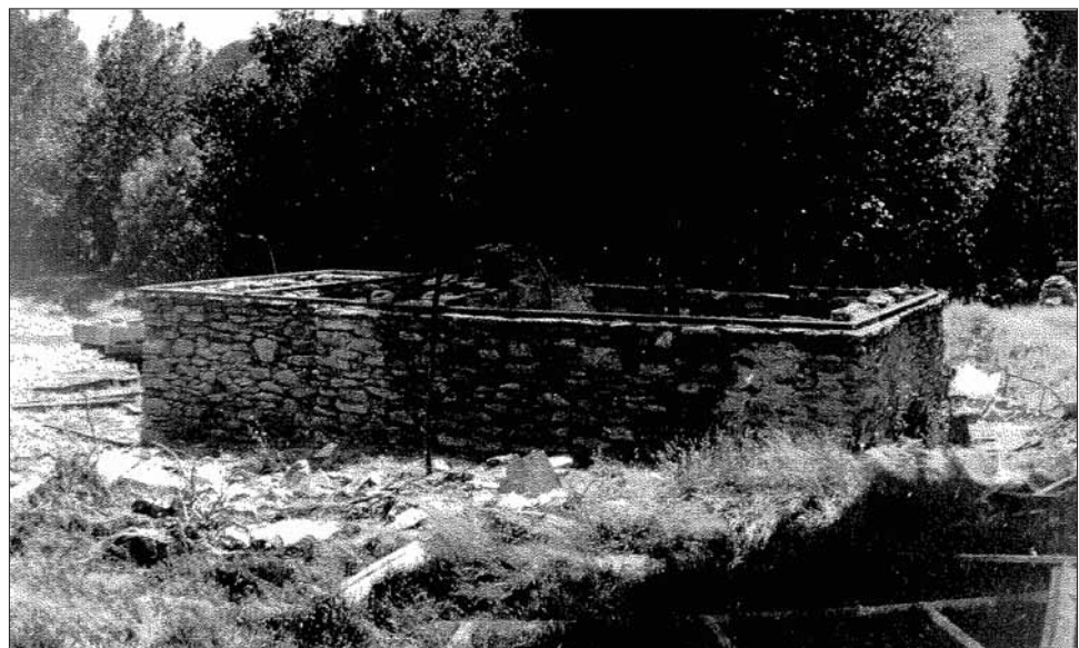
Figure 7. The Bakehouse (from south side) during restoration in the late 1970s. The front and back walls have been rebuilt.
