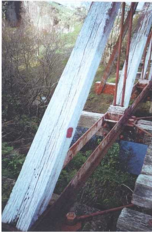
Figure 1 (top left). The distinctively whitish colour of components treated with Busan 30L is evident on this king strut at the Waikino end (component 7). The lower part of the queen strut in the background (5), treated with Boracol, was pale in colour but not distinctively different from the untreated section of the strut.
