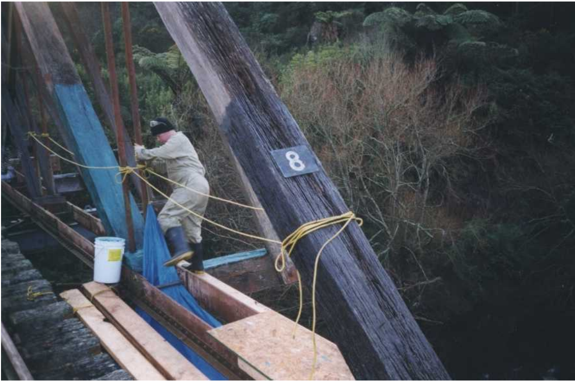
Figure 6. Components at the time of treatment. King strut 1 in the foreground has just been coated with CD50 and the tarpaulin installed to prevent spillage into the creek is being removed. Queen strut 3 and the top of transom 17, coated with CN Emulsion earlier in the day, are in the background.
