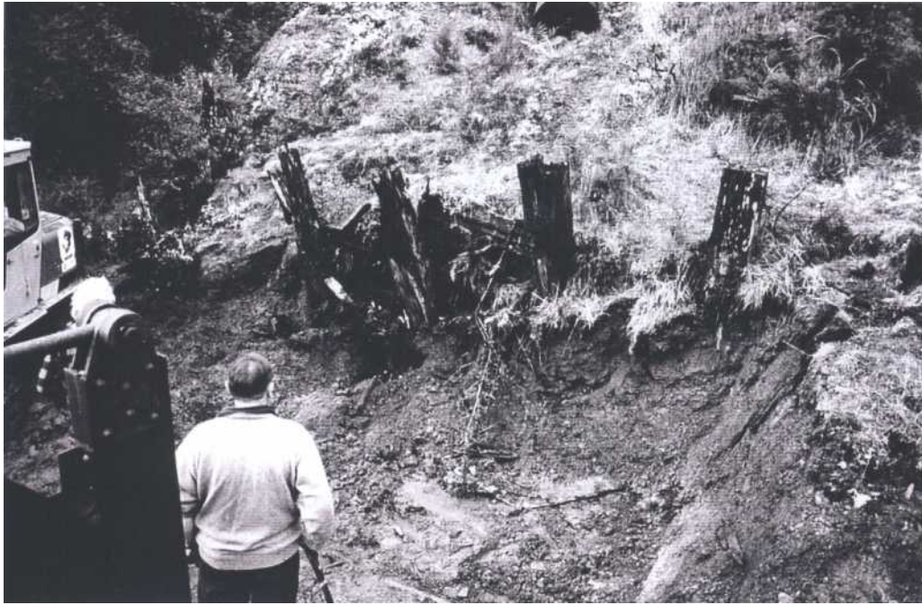
Photo 17: Remains of retaining wall.
