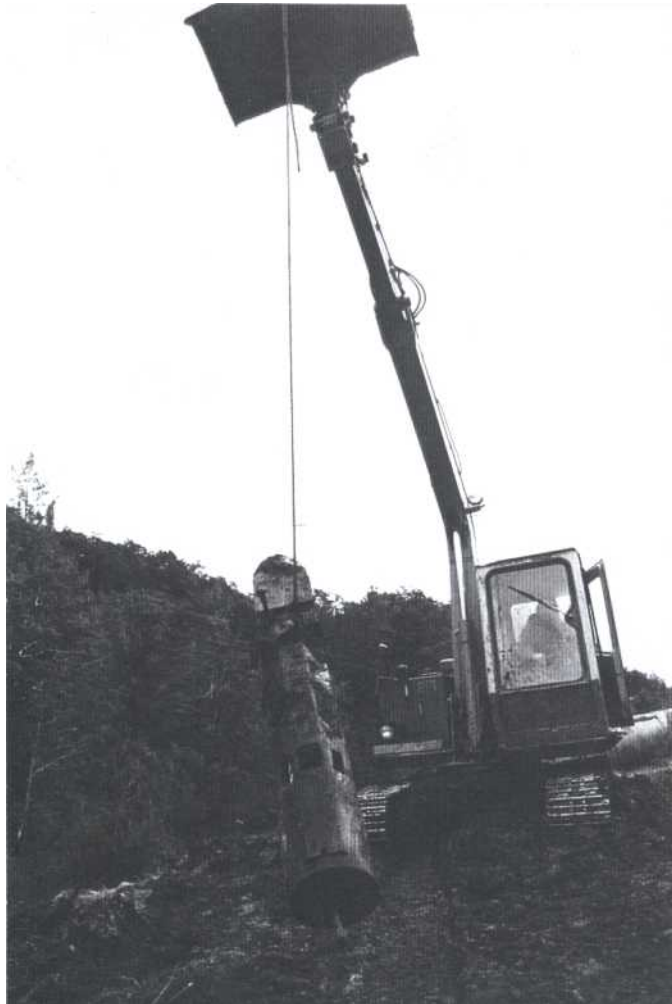
Photo 9: Hoisting whim spindle.
