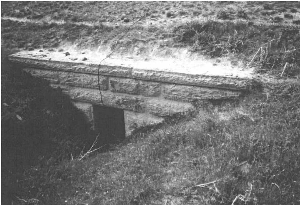
Figure 7. Examples of schist masonry, all brought to course. Upper left.:Poolburn tunnel 12. Upper right: a big arched culvert at Ida Valley station Below: a square culvert (98.48) and an arched culvert (98.39).
