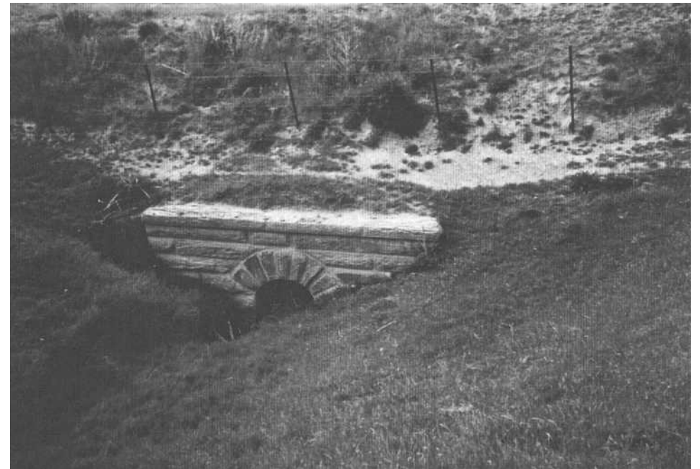
Figure 7. Examples of schist masonry, all brought to course. Upper left.:Poolburn tunnel 12. Upper right: a big arched culvert at Ida Valley station Below: a square culvert (98.48) and an arched culvert (98.39).
