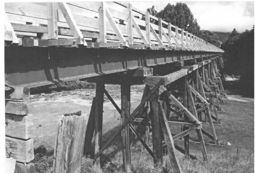
Figure 8 Bridges between Middlemarch and Clyde Upper left: a wooden trestle bridge over Gorge Creek (No.67). Upper right: Muddy Creek bridge (No.72) with RSJs. Lower left: Manuherikia No 2 bridge. Lower right: Muttontown bridge.
