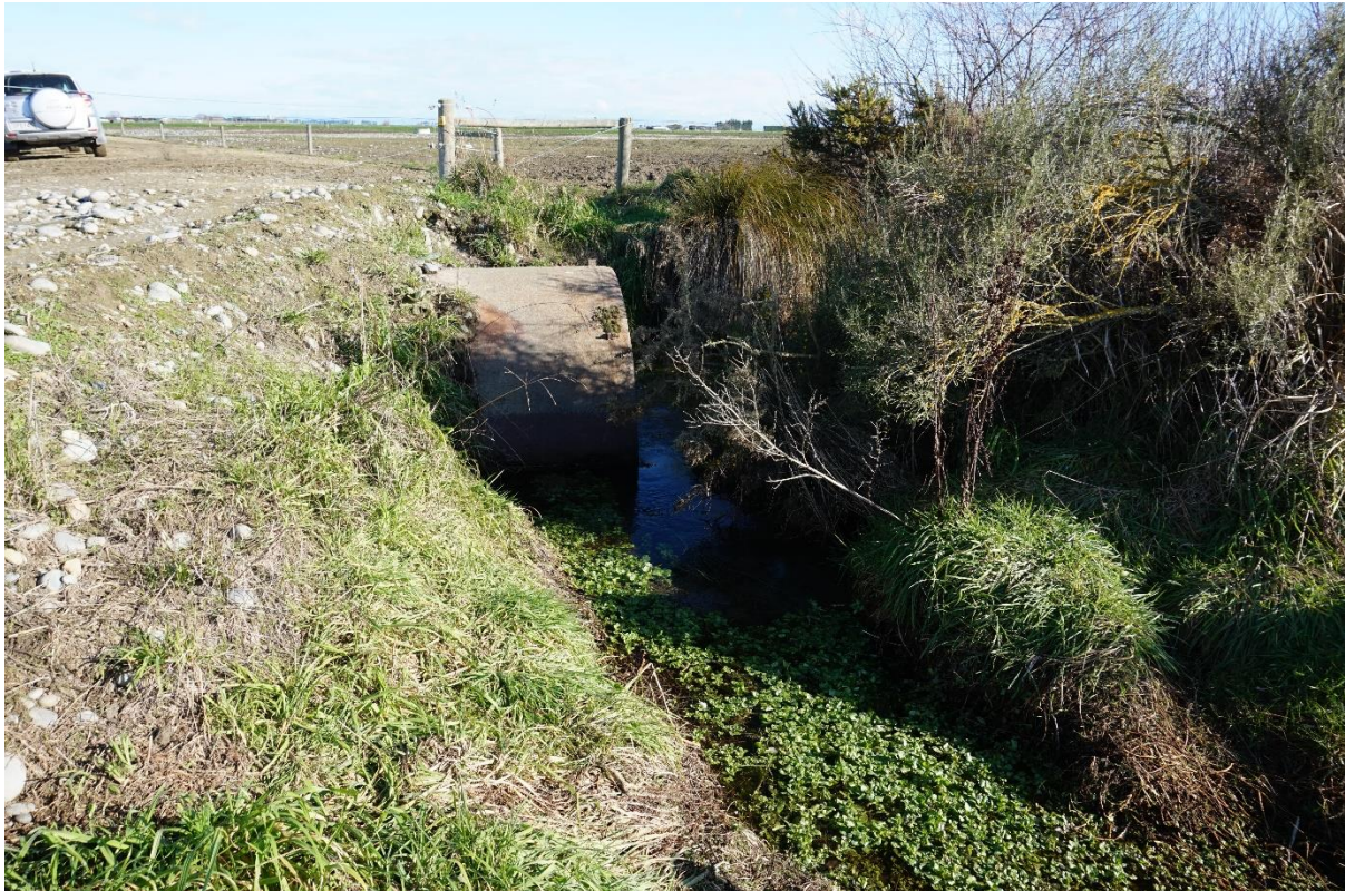
Plate 3: A culvert located downstream of the large willow wetland. This culvert is likely acting as a barrier for indigenous freshwater fish passage. 8 July 2021.
