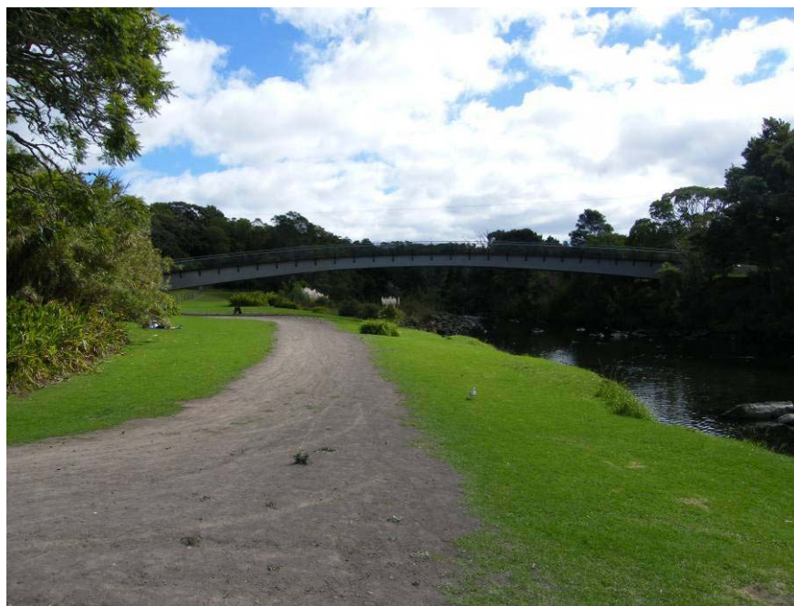
Kereikeri Basin Footbridge: Photo Terry Conaghan
