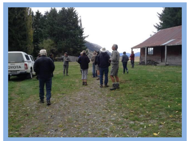
St James Station Buildings
