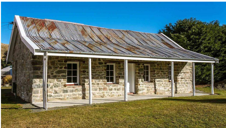
Hakatere Station buildings (Image: Department of Conservation)
