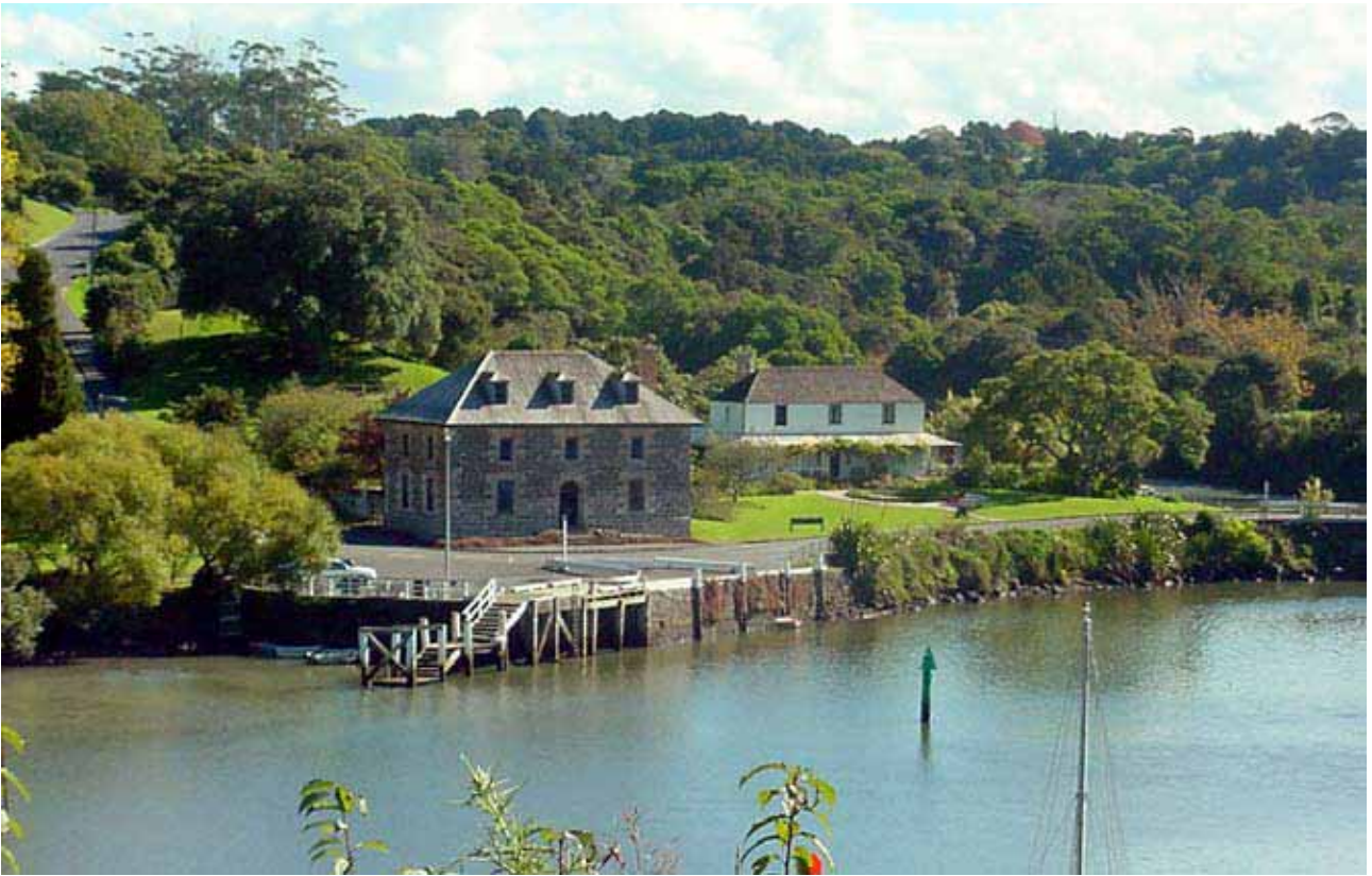
Stone Store, Kemp House and wharf. Otwyn Crutchley
