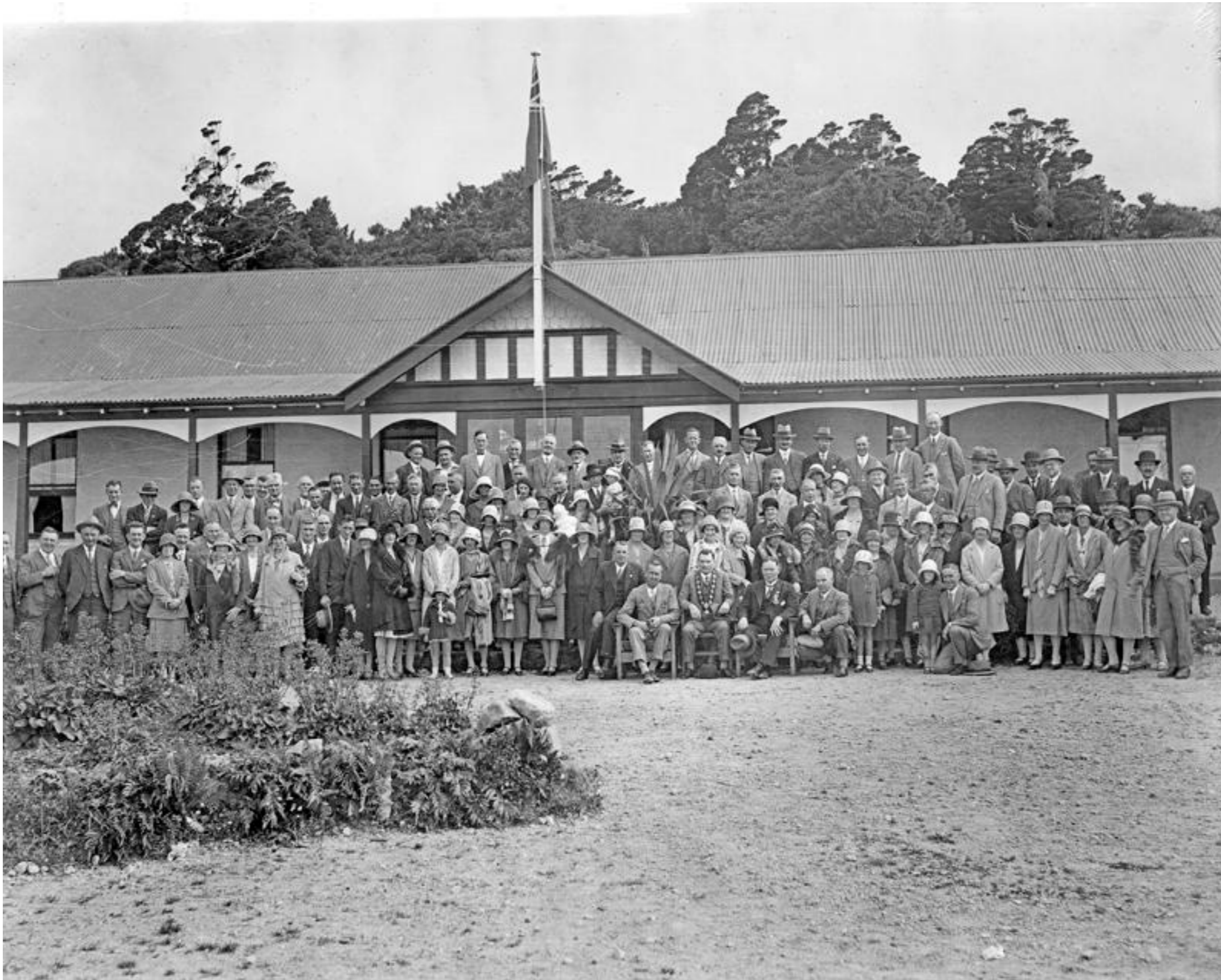
Figure 26: c.1923 photograph of the North Egmont Hostel, showing a flagpole erected on the central gable front (Puke Ariki: WD.009803).
