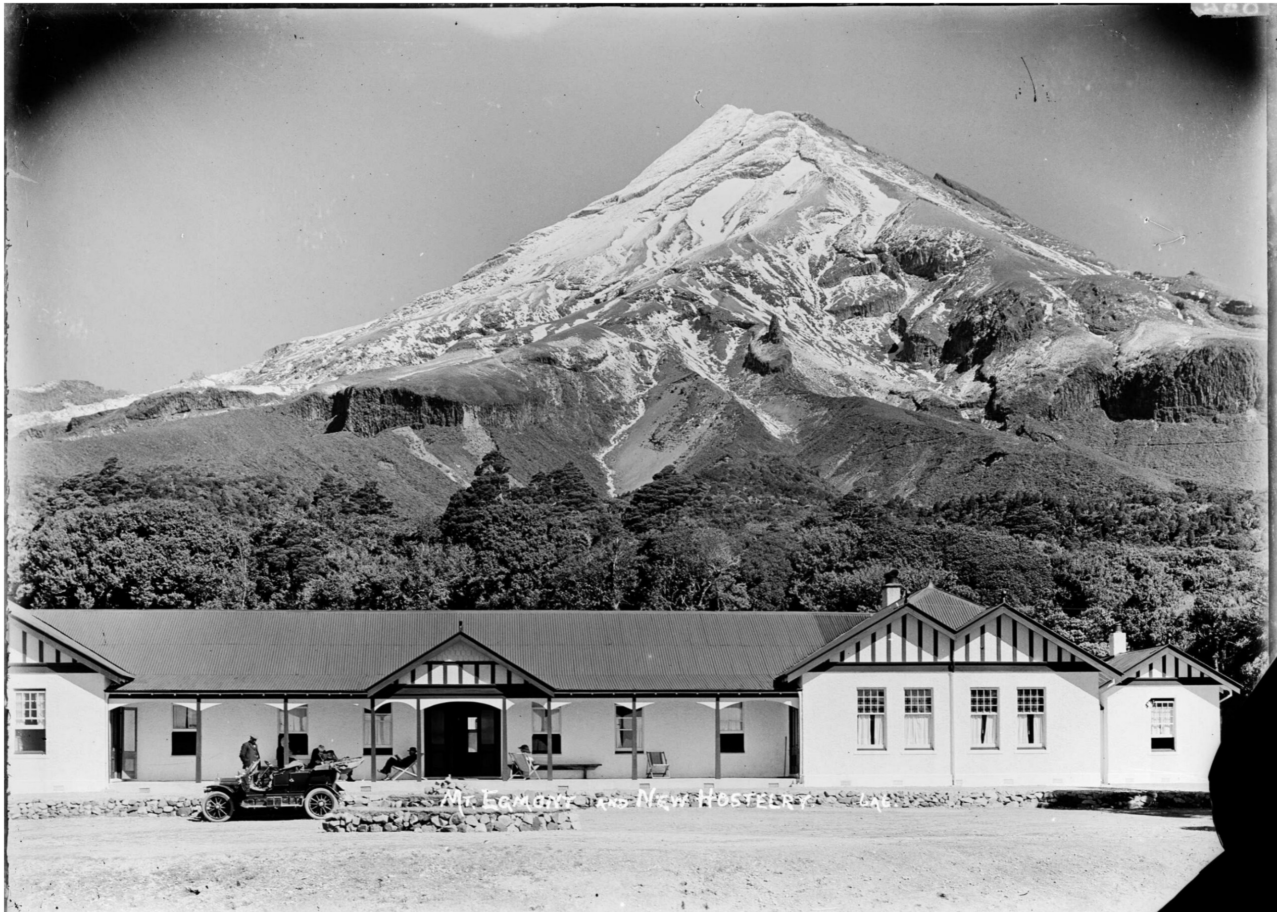
Figure 23: c.1910s photograph of the North Egmont Hostel (ATL: PA-Group-00719).
