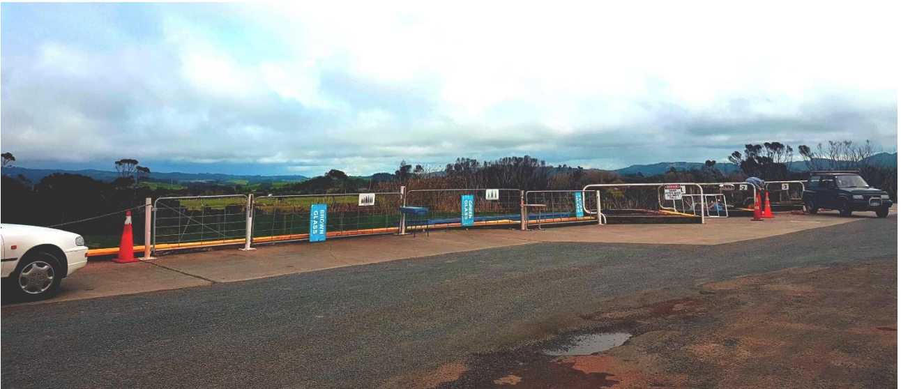
Figure 1: Refuse Transfer Station Disposal Area
