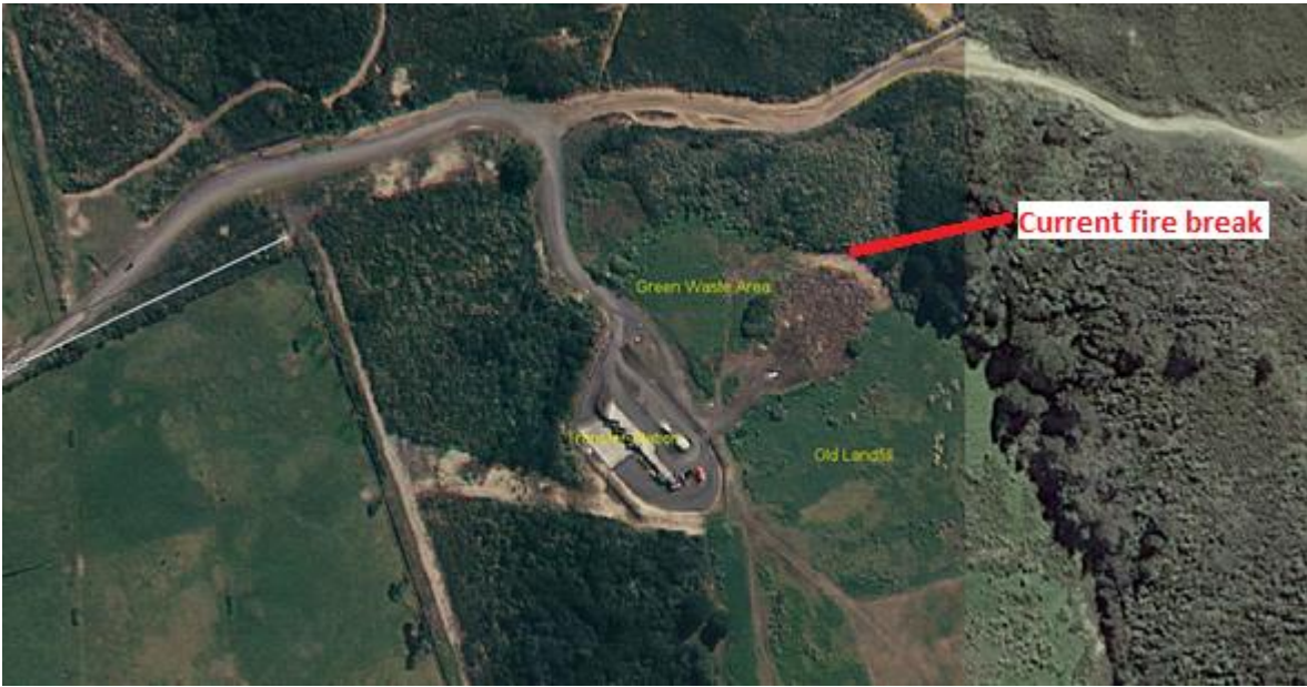
Figure 5: Current Fire Break
