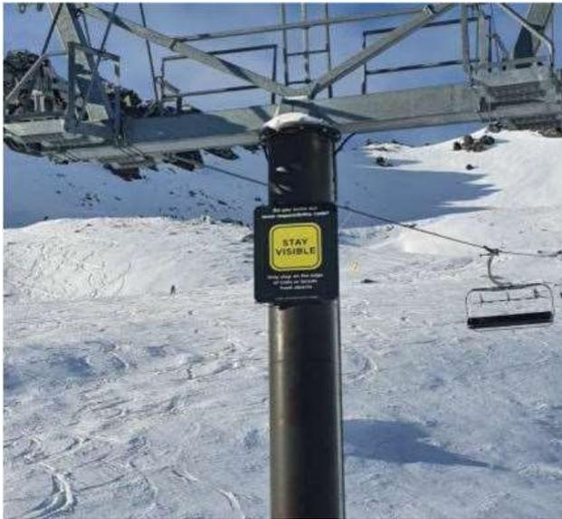
Figure 8: Example of paint colour and galvanised “head” structure from Application
