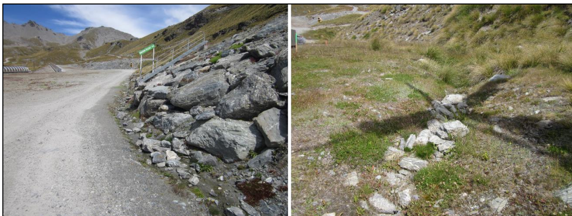
Plate 7: Left: overland flow path at the toe of the rock wall. Right: Overland flow path at the toe of the tussock grassland slope.
