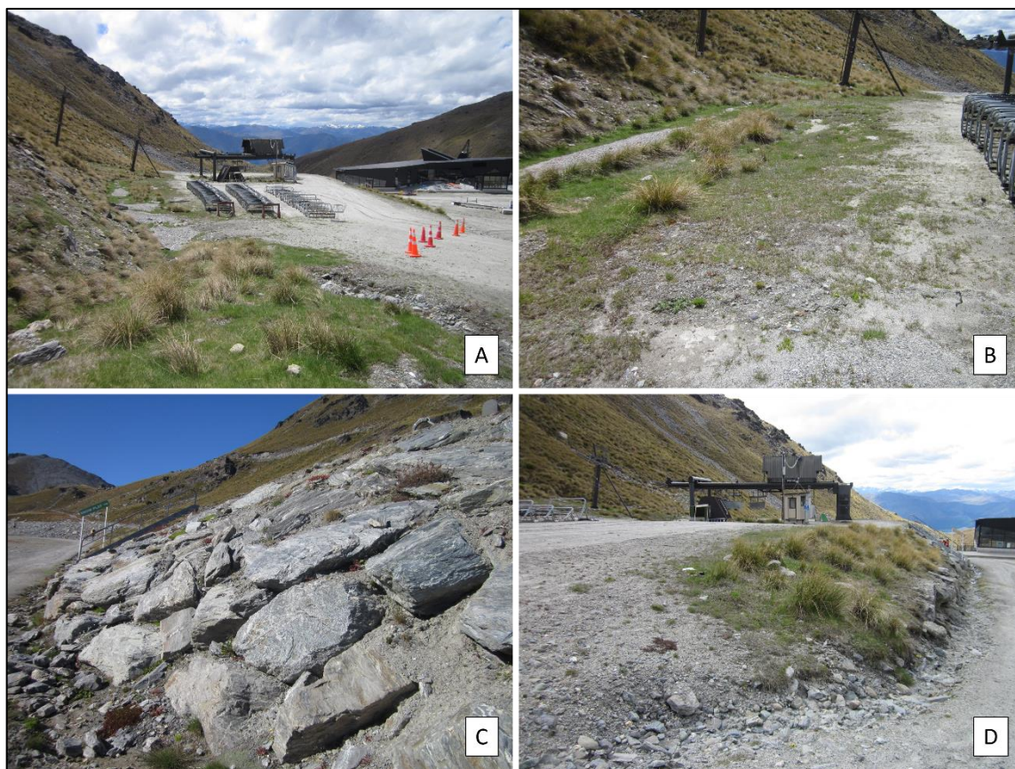
Plate 5: Photographs of the Lower Lift station location. A – general overview. B – photograph showing general cover of disturbed areas. C – northern end of the rock wall. D – Southern end of the rock wall.
