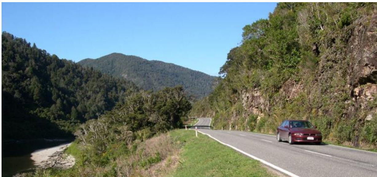
Plate 14: Steep cut batters on the Lower Buller Gorge reduce the area of native vegetation removed by the road; this is balanced against the reduced ability to establish a dense vegetation cover (photo taken 2011).
