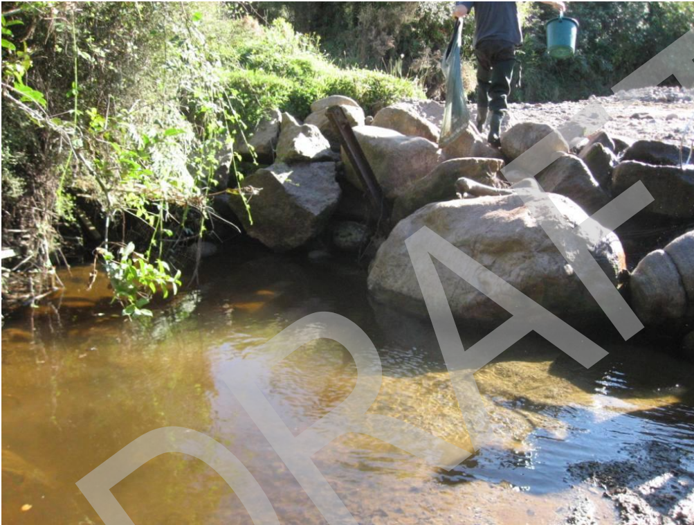
Figure 18: Partial fish passage barrier on West Creek at the Nine Mile Road ford.
