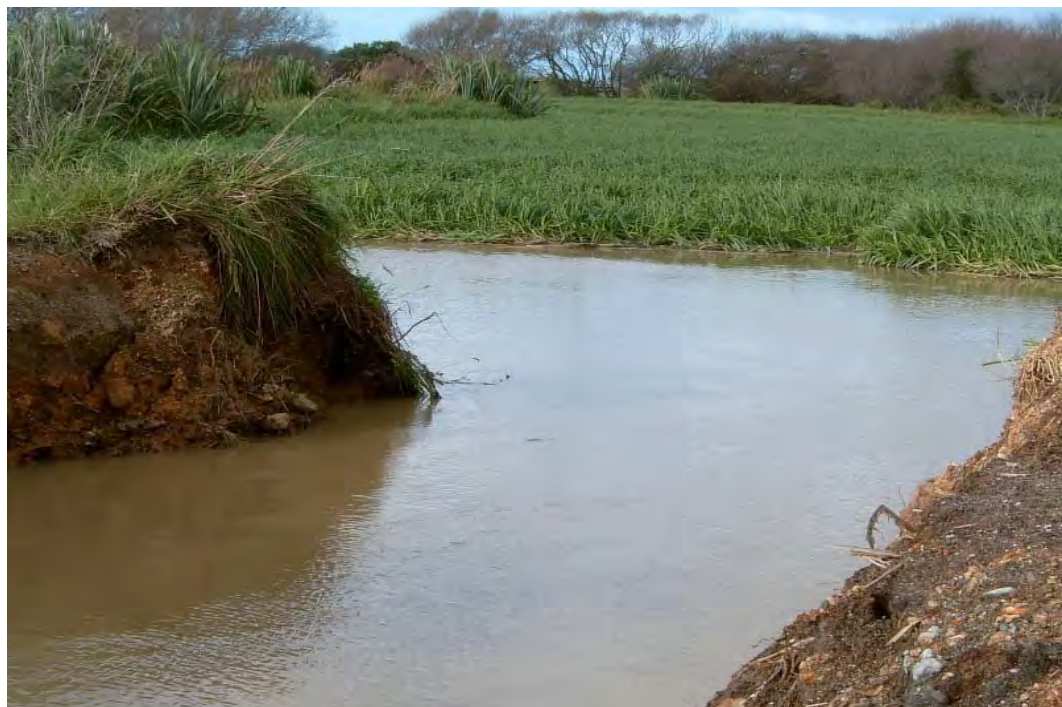
Figure 9. Embankment breached at eastern end of the eastern lagoon near Tarawera River. Water sweetgrass ( Glyceria maxima ) infestation beyond (Ian Smith, 31 May 2005).
