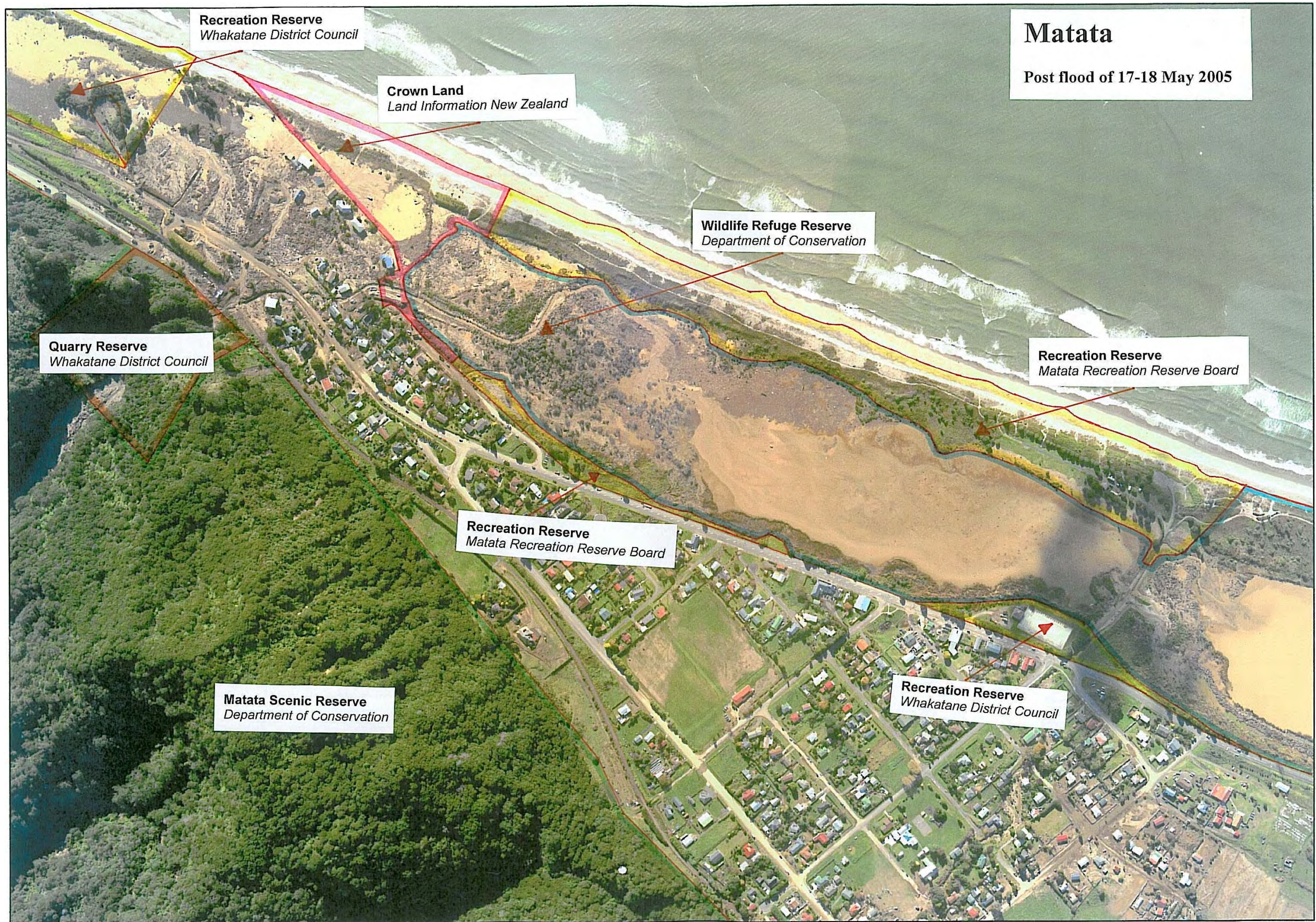
Figure 7. Aerial photograph of western lagoon, Matata, immediate post flood of 17-18 May 2005.
