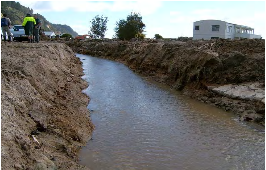
Figure 10. Awatarariki Stream outlet looking upstream (Ian Smith, 31 May 2005). Note, the stream has been channeled into a narrow cut flowing directly towards the remnant area of the western lagoon.
