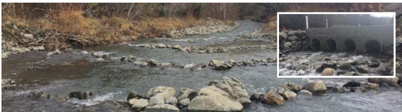
Backwatering established downstream of culverts to raise the water level and ensure no perching of culverts and good passage upstream and downstream from the culverts. Inset shows downstream view of culverts with backwatering in place so no perching.
