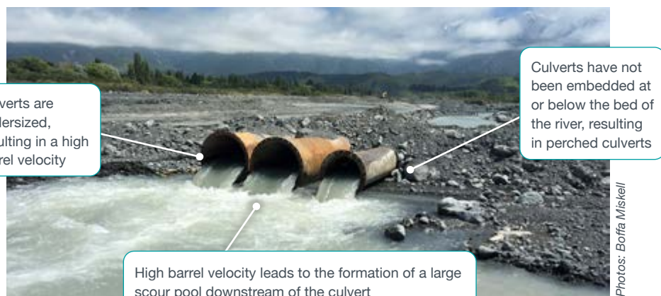
An example of temporary culverts that do not provide fish passage.
