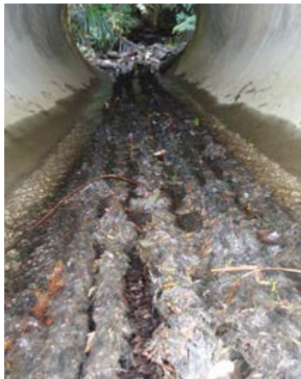
Mussel spat rope installed within the base of a culvert to help fish passage through a culvert.
