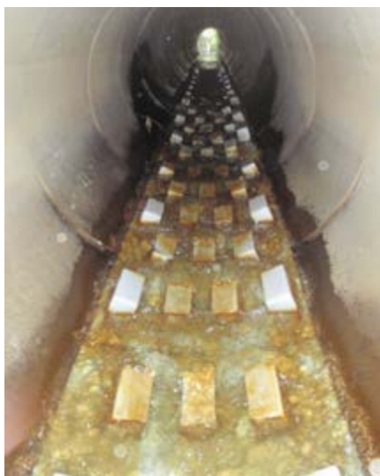
Spoiler baffle sheet installed into the base of a culvert to help fish passage through a culvert.
