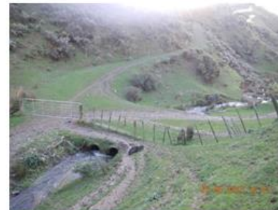
Structure 9: Culvert inlet looking downstream
