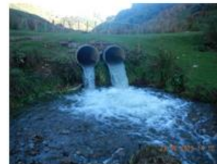
Structure 9: Culvert outlet looking upstream
