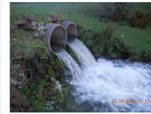
Structure 9: Culvert outlet looking upstream
