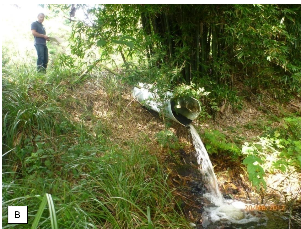
Figure 1: A,B. Poorly installed culverts on a tributary of the Mangakotukutuku stream in urban Hamilton. In the lower example a perch height in excess of 1m combined with a 12m pipe length and pipe gradient in excess of 10 makes this a formidable barrier to even the most aggressive upstream climbing species.
