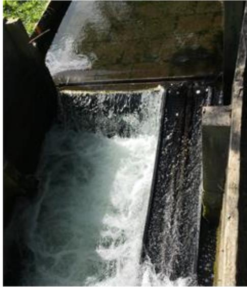
**Figure 1: The floating fish ramp (with spat rope) on the Irongate Stream weir**
