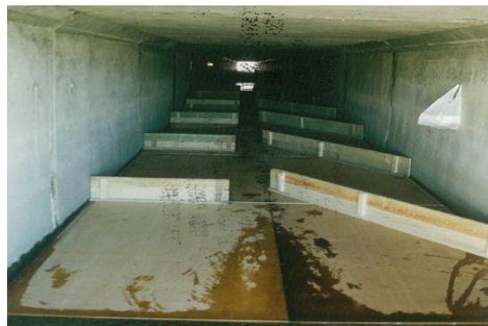
Figure 3. Baffles on a 5% gradient base overlying the culvert with a 2% gradient base. (Source: M Webb)
