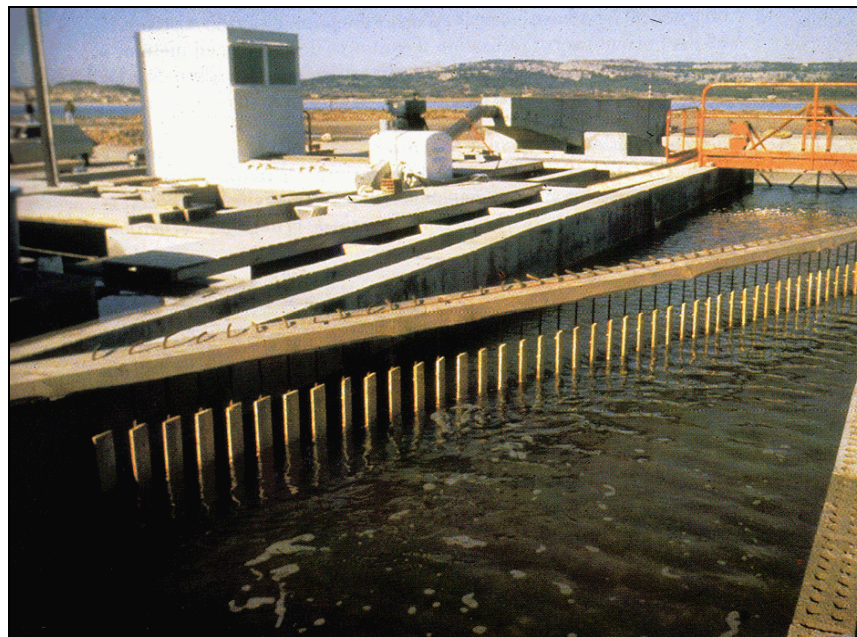
Figure 16 : Experimental louver arrangement, Gruissan, France (photo M. Larinier).
