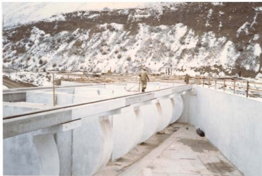
Figure 4: Large drum screens during installation, Washington, USA
