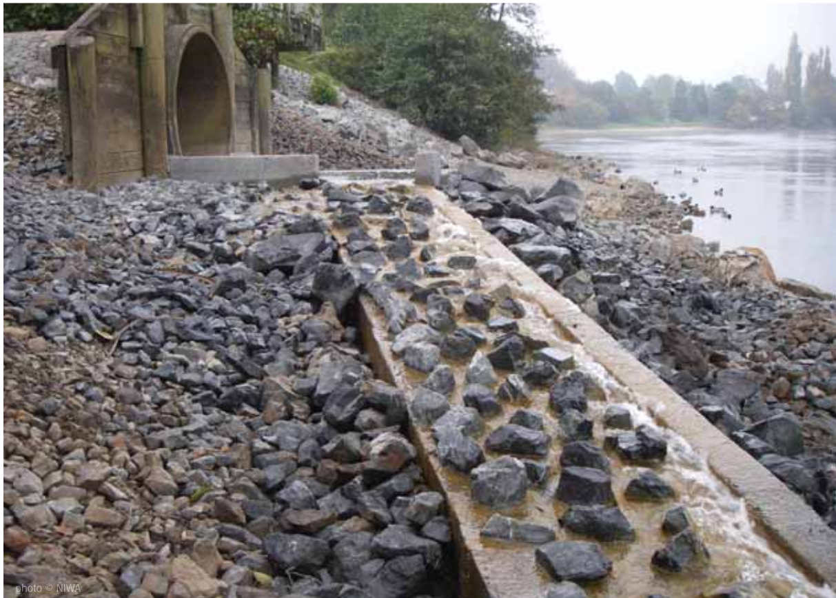
FIGURE 10 An example of a remediation solution for a perched culvert. A rock ramp and receiving pool were installed at the end of this culvert in Hamilton to provide upstream access for smelt and inanga. Monitoring showed that while fish were now reaching the bottom of the culvert, they were not able to pass through the culvert due to its length and high water velocities. Following installation of baffles in the culvert, monitoring showed an increase in the abundance and diversity of fish upstream of the culvert (Franklin & Bartels 2012).
