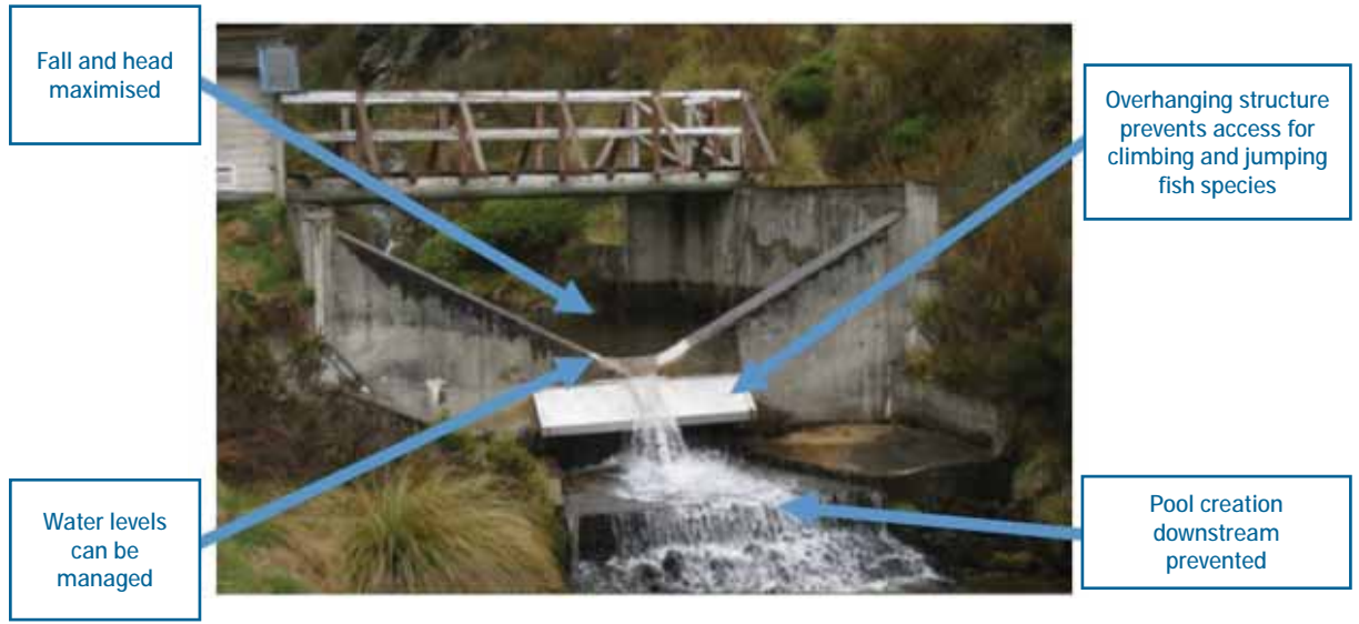
FIGURE 2: Example of a weir that has been installed to intentionally prevent invasive species passage.
