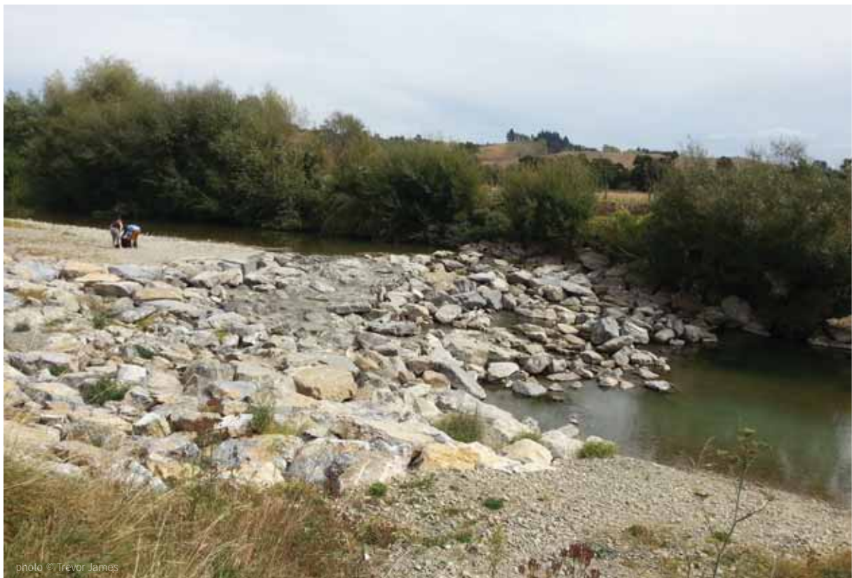
FIGURE 6: This weir was constructed with large boulders in a medium-size river (annual flood flow of 180 cumecs). This structure was found to be a barrier to common smelt and inanga. Several thousand common smelt were recorded below the weir but only three were ever found upstream. The highly turbulent flow between the boulders appeared to be the cause of the restriction to these fish. The first option used was to pack 20–50 mm crushed rock material between the boulder but that got reamed out by floods. After this it was felt that concrete was the only option (given that the basic structure had to stay). The photo is of the weir with a lower gradient (zig-zag) concreted ramp installed. In building the ramp 4 m 3 of ‘manhandlable’ angular rock was slotted in all the larger voids and 4 m 3 of 30 MPa 8 mm block fill concrete was used to build the ramp. We are yet to do a fish survey to confirm that this rock ramp has been successful at providing fish passage.
