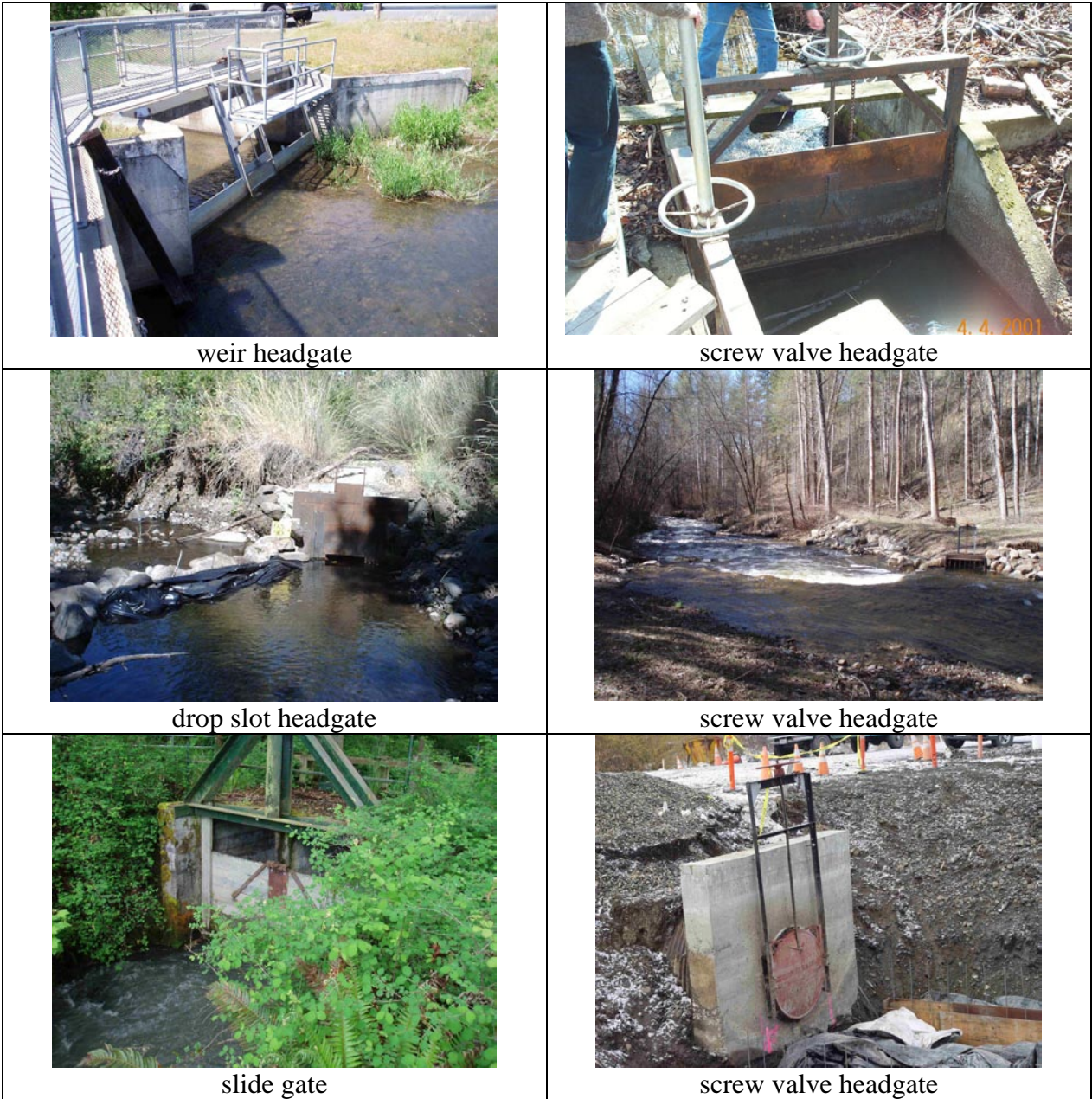
Figure 8.1. Examples of common headgate styles.
