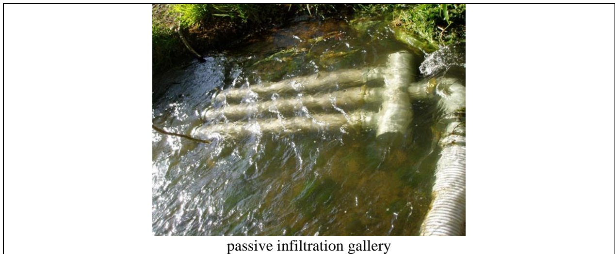
Figure 8.11. Photo example of passive infiltration gallery
