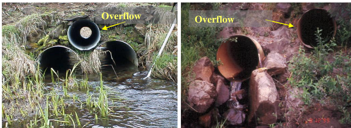
Figure 3.1. Examples of overflow culverts.
