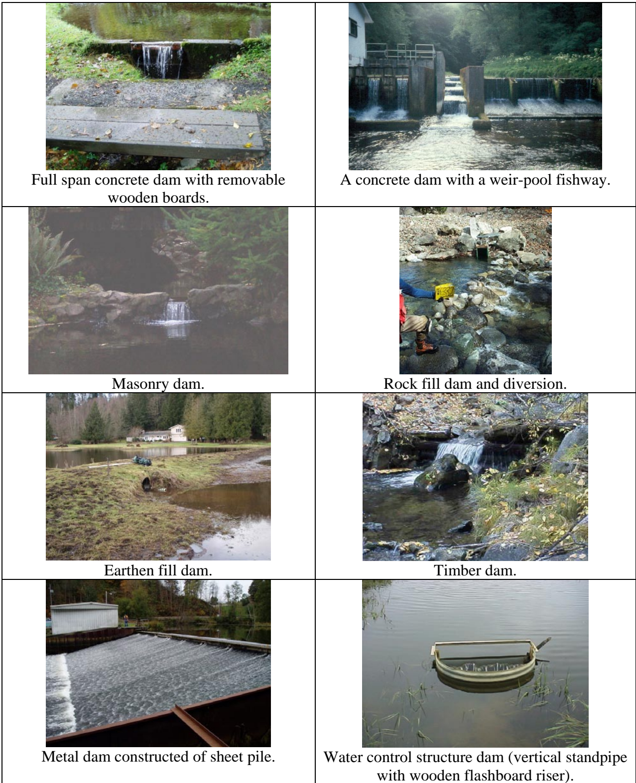
Figure 4.1 Photo examples of dam structures.
