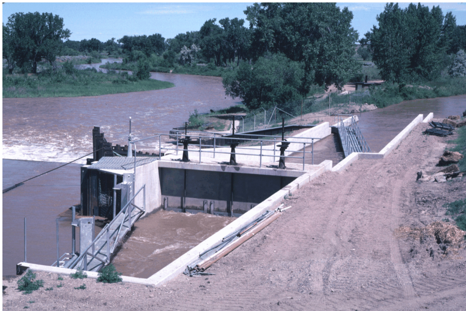
Figure 116.—Overview of T&Y Diversion with fish louver structure – Example 4 (T&Y Irrigation District).
