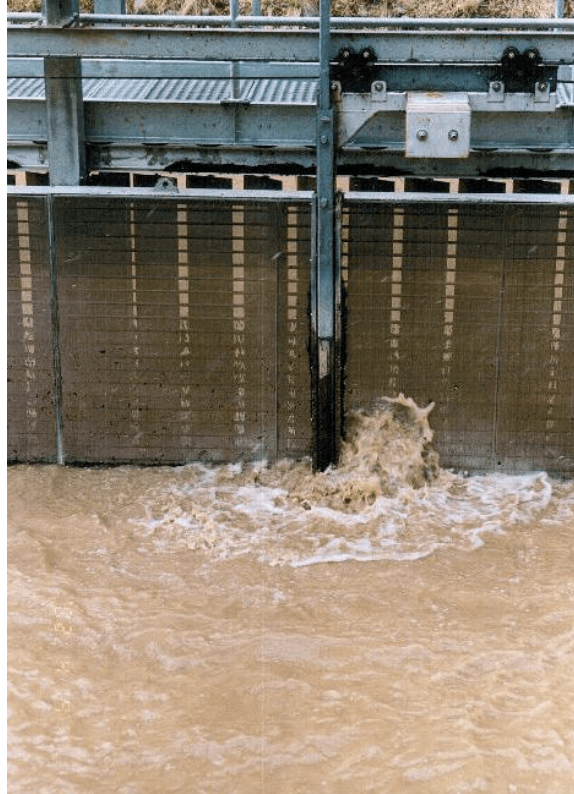
Figure 66.—Flat plate screen with horizontal brush cleaner and air nozzle at bottom of cleaner arm.
