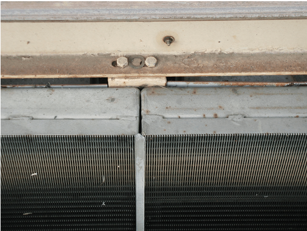
Figure 63.—Joint with caulking – Red Bluff flat plate screen (screens bolted to supports).
