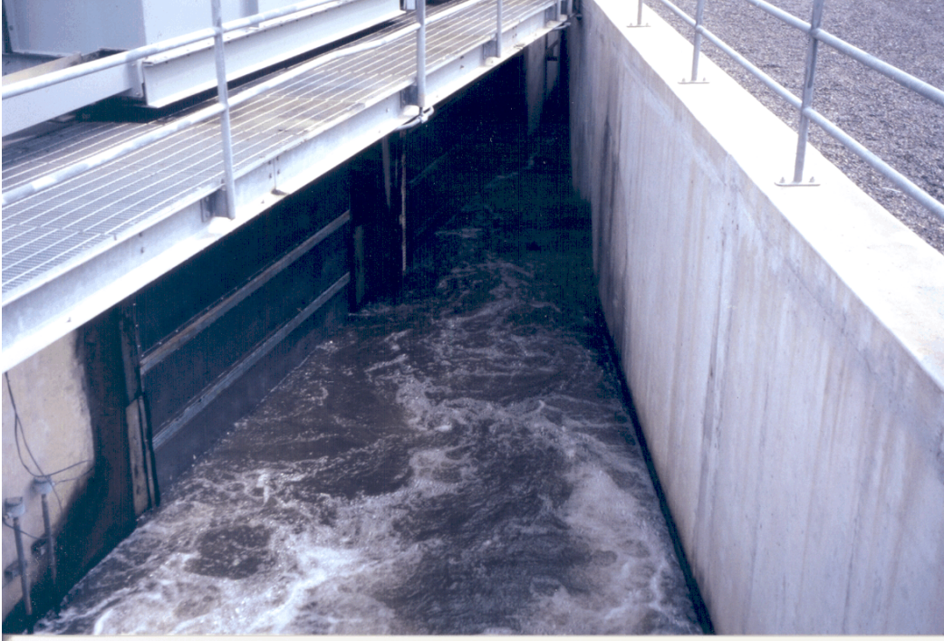
Figure 76.—Traveling screen field site with angled wall – Chandler Canal secondary screen/pumpback structure.
