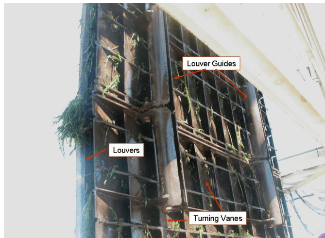
b. Looking at downstream side of removed louver.
