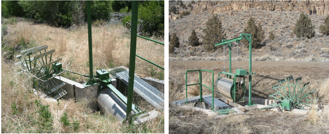
a. Operation – in the dry.
