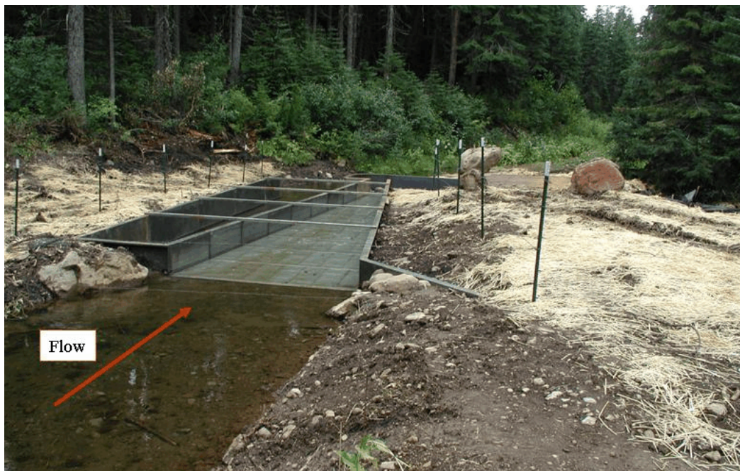
Figure 20.—Horizontal flat plate screen, East Fork Ditch Company, East Fork, Weiser River, Idaho.
