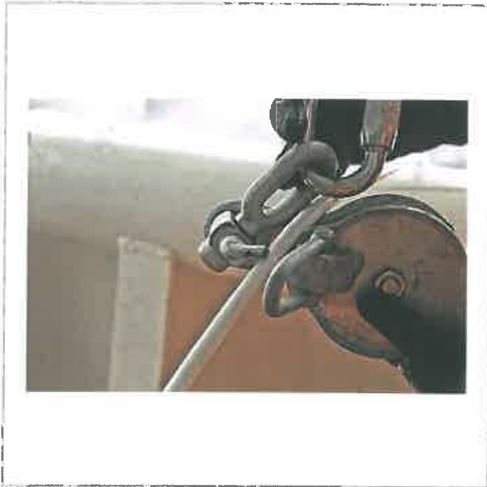
Opening pulley block to insert PAM cable
