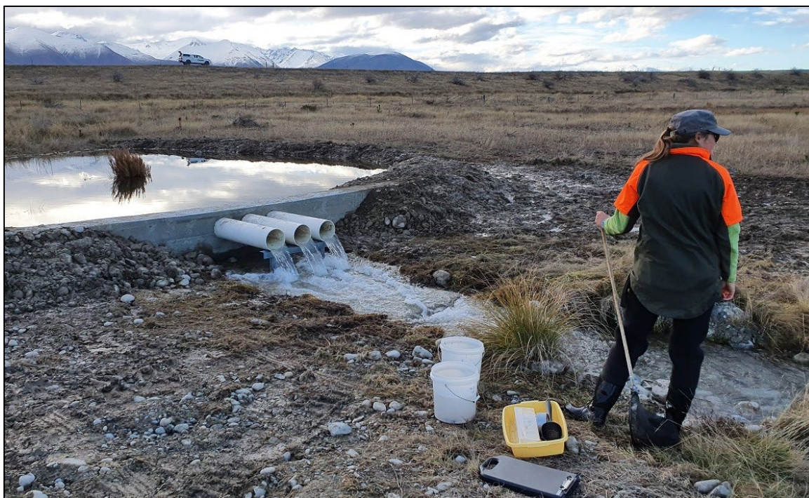
Figure 11. New perched culvert trout barrier to protect bignose galaxias in Waterwheel Wetlands spring fed stream. Photo: Dean Nelson
