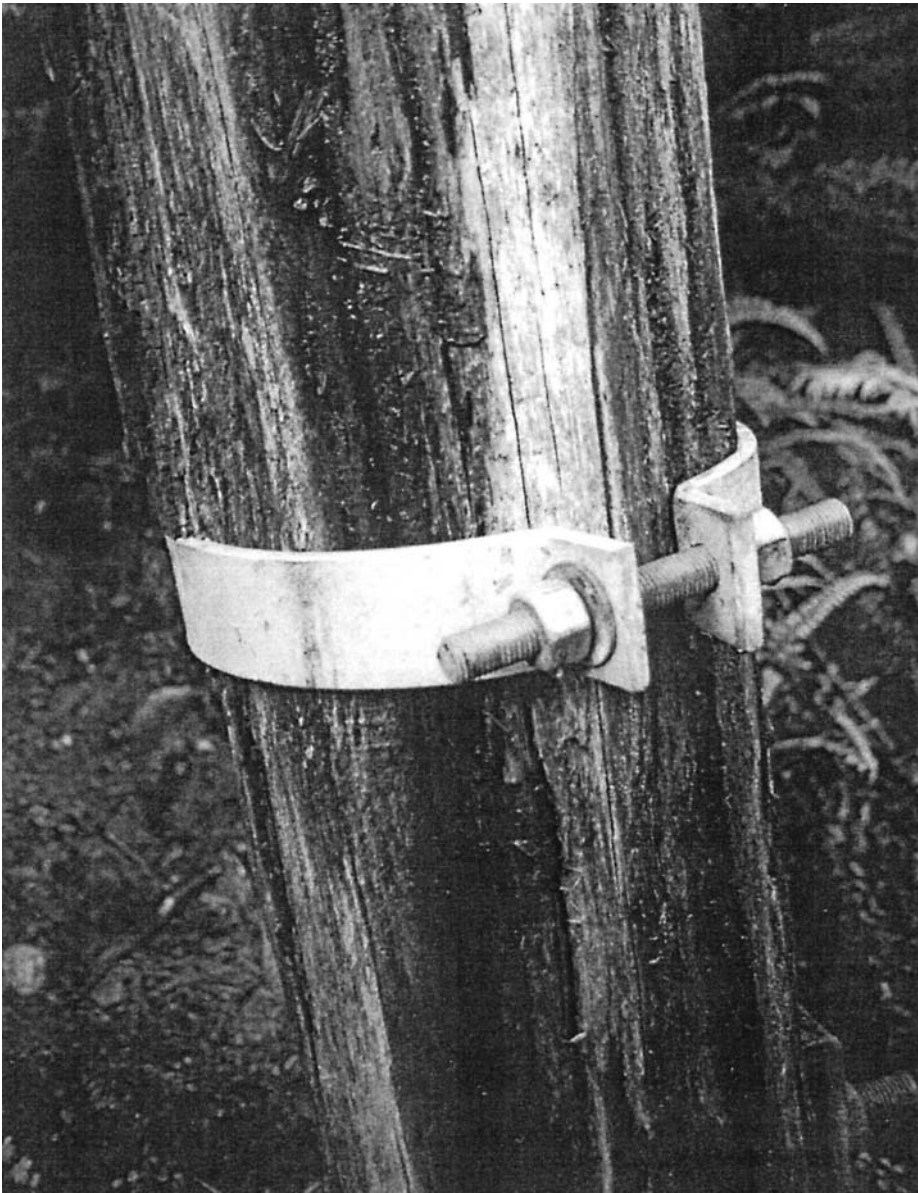
Fig. 13: Steel clamp on splintering pile. Sandhill viaduct, Port Craig.
