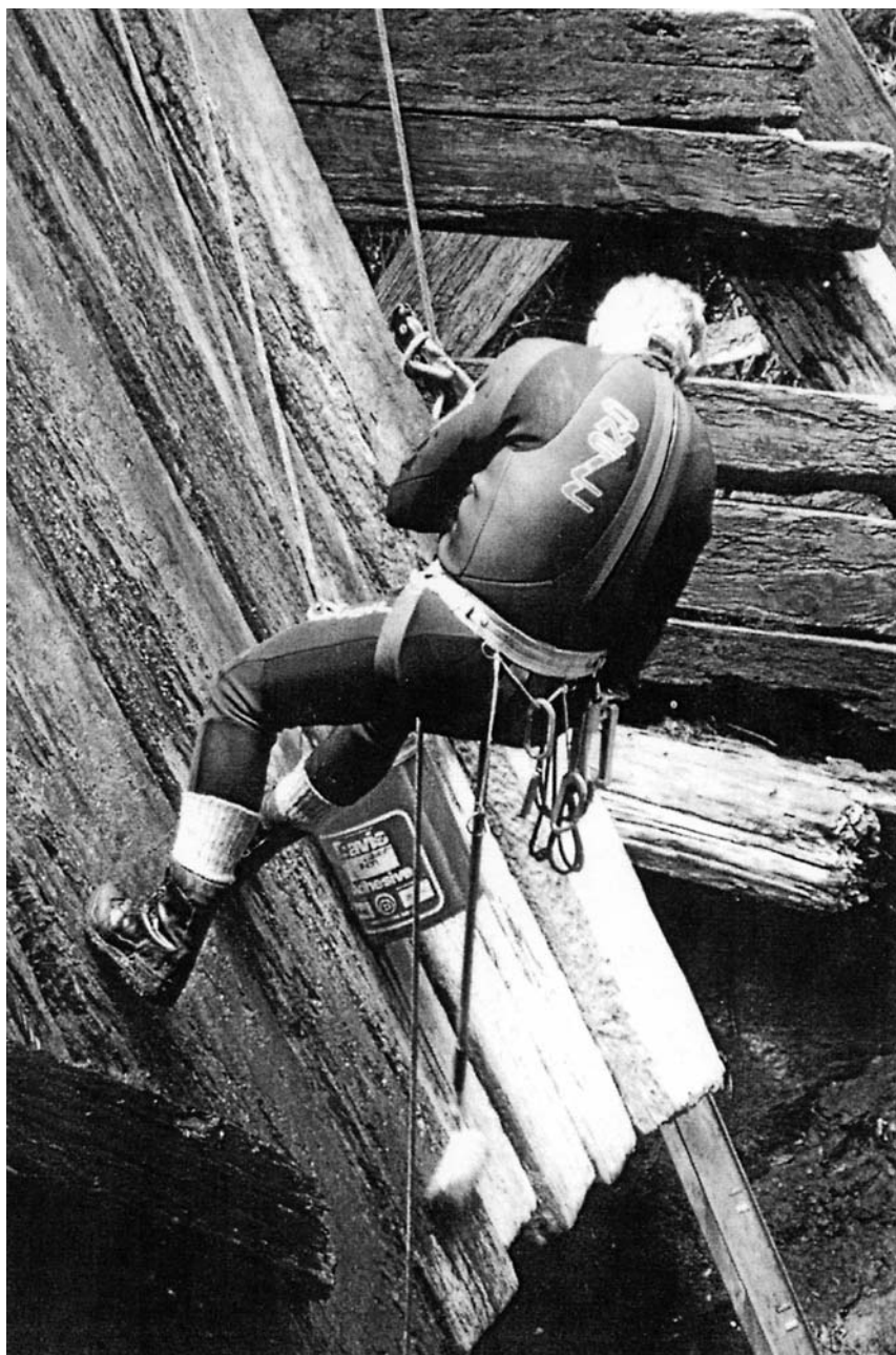
Fig. 14: Applying CD50 to Christmas Creek dam. Note wetsuit, abseil gear and long handled roller. Working below one's own body minimises risk of contact with preservative.
