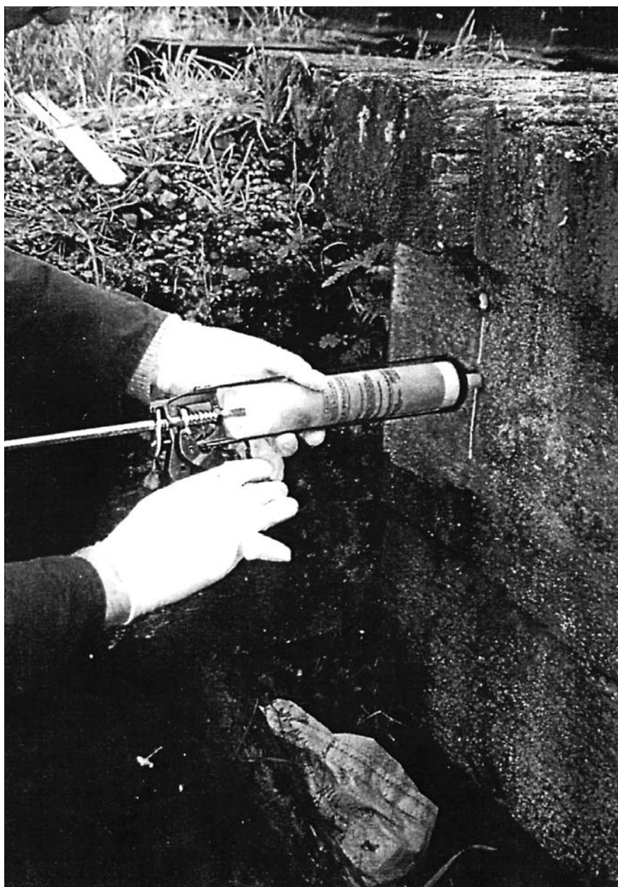
Fig. 18: Injecting Polegel with a caulking gun.
