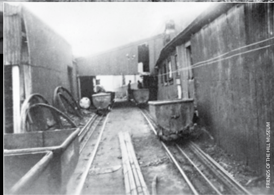
The rope road passed right between the workshops and associated sheds. The view on the next page looks the opposite way, across the top of the fitters' shop. Full coal tubs weighed 11–12 cwt.
