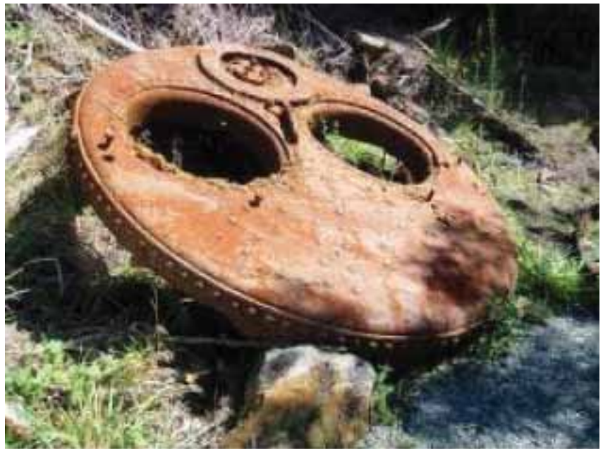
A Lancashire boiler endplate is all that remains of the boilers. As it is smaller than the usual 8' diameter for such a boiler it is believed to be the remains of 701/3977, the 20hp AW Smith of Glasgow boiler, first inspected at Blackball on the 22 February 1902.
