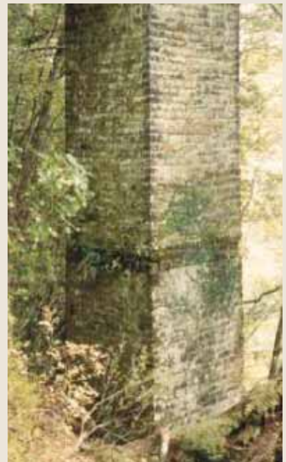
Top: 1892 wooden chimney site, rebuilt in 1897 in brick. Below :second chimney base, built in 1895, extended in 1896—dark lines represent the original height. JIM STATON COLOUR PRINTS
