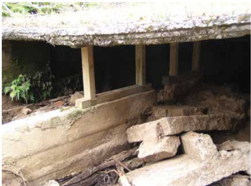
1904 Capel fan return airway opening, the fan itself was sited centrally in front of the opening, with air doors both sides of the fan. JIM STATON, MARCH 2008
