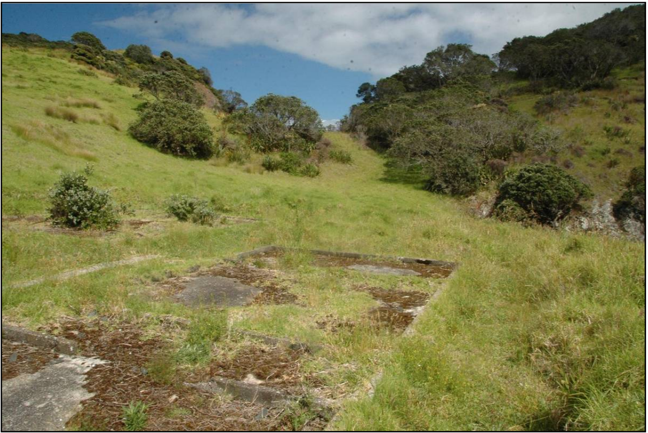
Appendix 3: A section of the campground foundations located on the bay flats (DoC).
