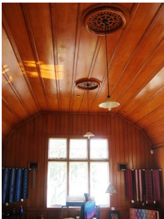
Figure 2: Kauri interior with curved ceiling and elaborate fretwork air vents (now used for light fittings) (left); Figure 3: detail of brass air vents on wall (above) (photo credits: Carolyn Smith).
