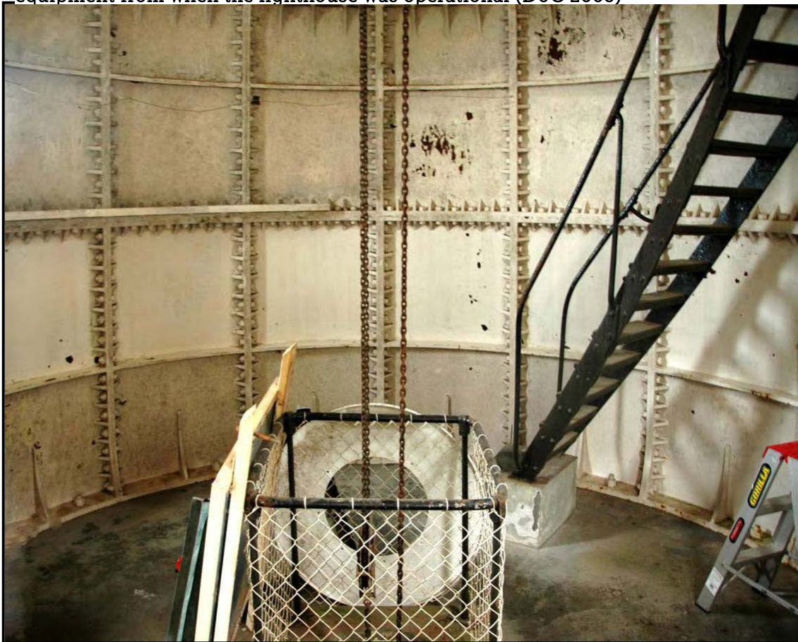
Appendix 4: The bottom floor of the lighthouse (DoC 2008)
