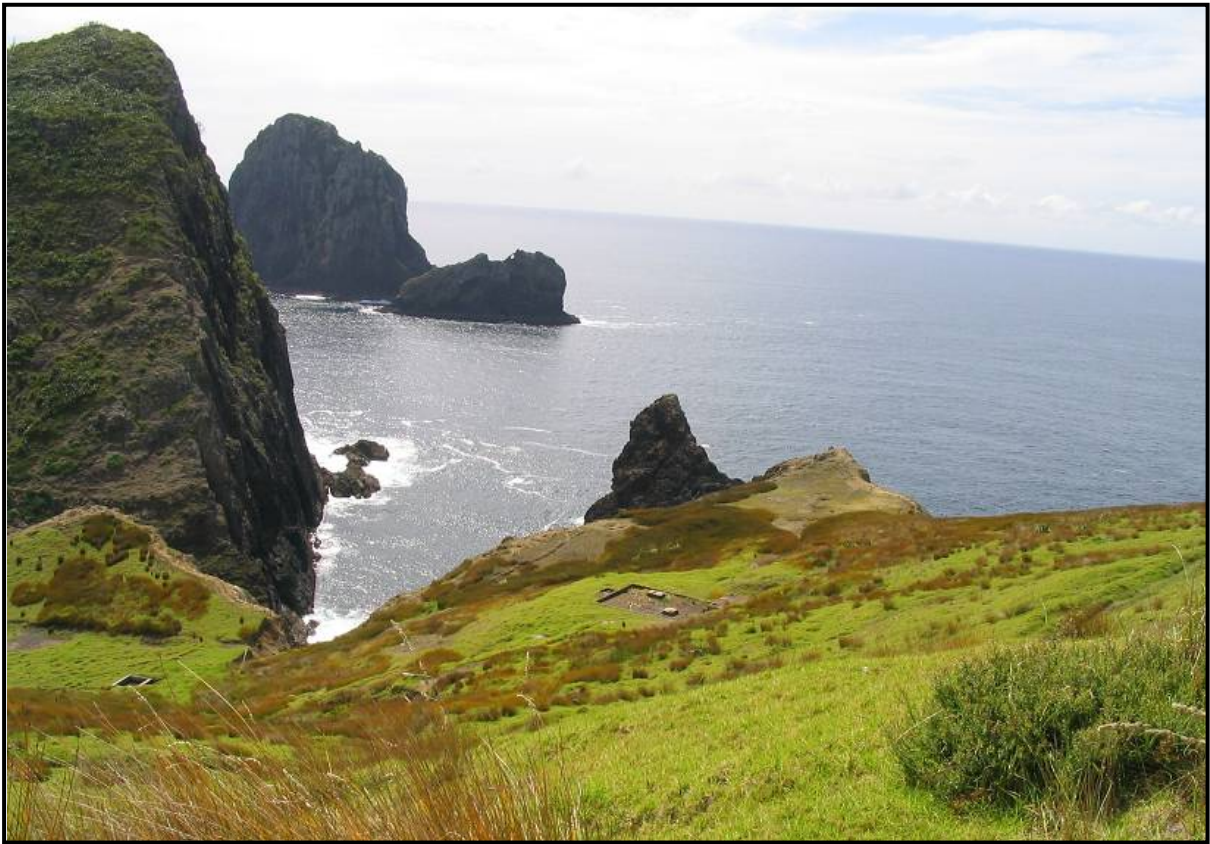
Appendix 7: The concrete pads from the second assistant keepers house (K Upperton 2010).
