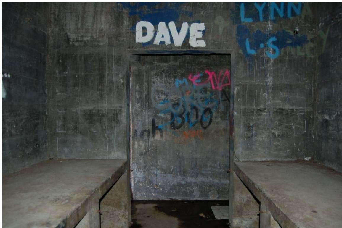
Figure 6: Interior of gun emplacement, showing shell recesses and bench for magazine racks above. Metal brackets for attaching shell recess doors are visible.
