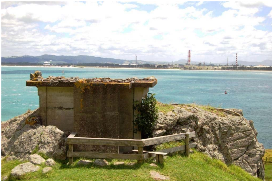
Figure 1: The rear of the B.O.P. Note the rocks cemented to the roof.
