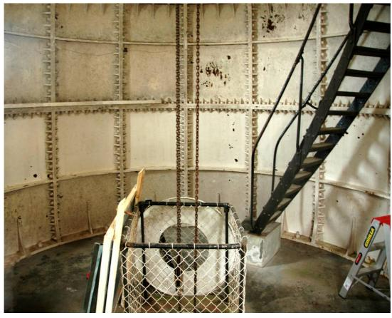
Figure 195 – The bottom floor of the lighthouse during cleaning. Here the flaking paint has been scraped, the floor swept and one row of panels has been scrubbed, 2008.
