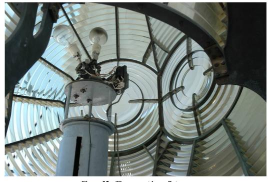
Figure 25 – The current lamp fixture.
