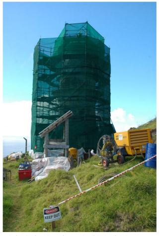
Figure 34 – The worksite during the paint work with the lighthouse covered in scaffolding.
