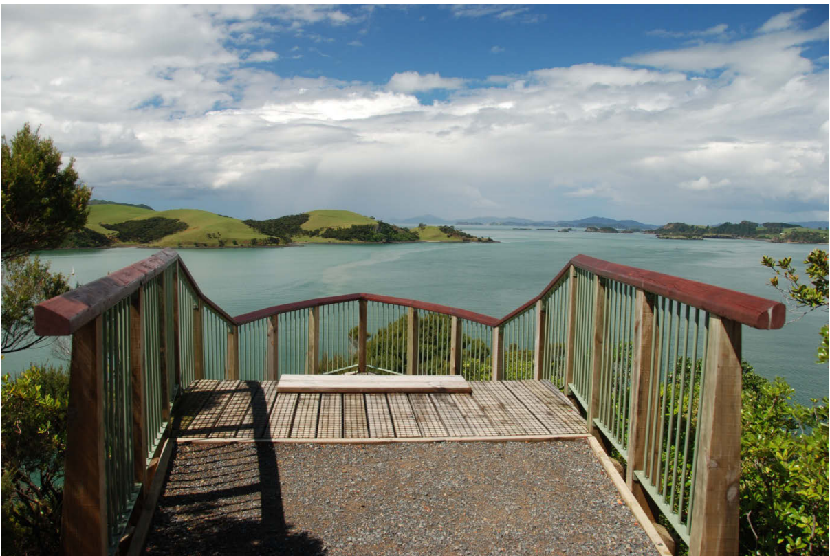
Figure 12: Viewing platform at end of Tareha Pa.
